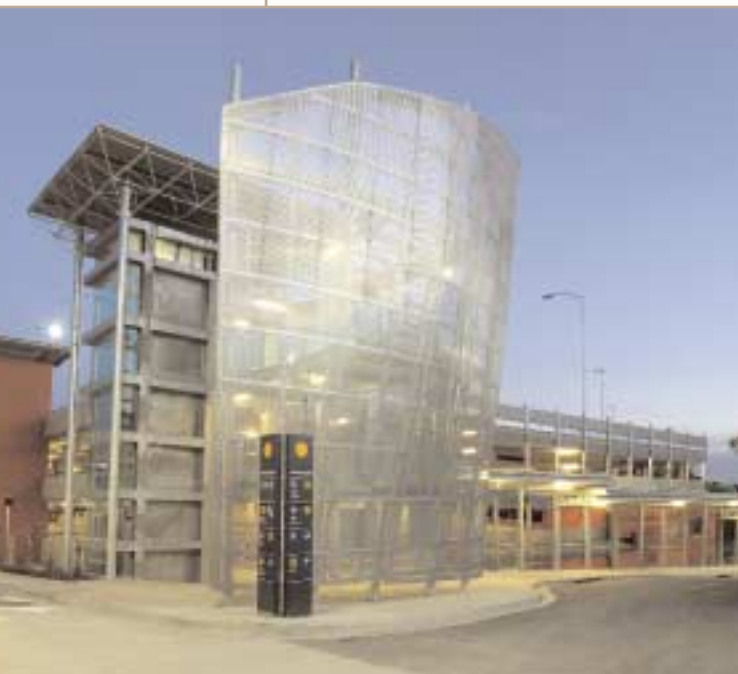
HOLSWORTHY COMMUTER CAR PARK
