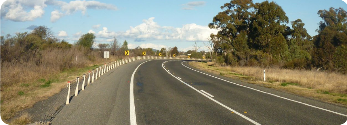
Wire rope safety barrier on road curve near Trewilga
