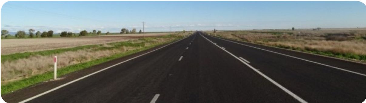
Intersection with Newell Highway at Grong Grong
