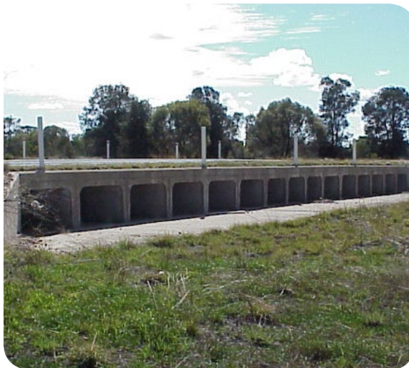
225 cell box culvert north of Moree
