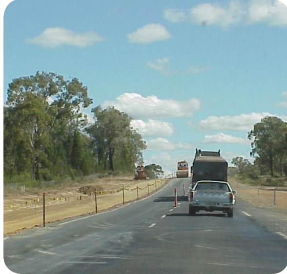
Pavement widening road works at Yarrabah
