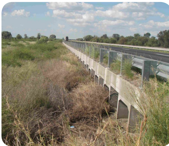
225 cell box culvert north of Moree
