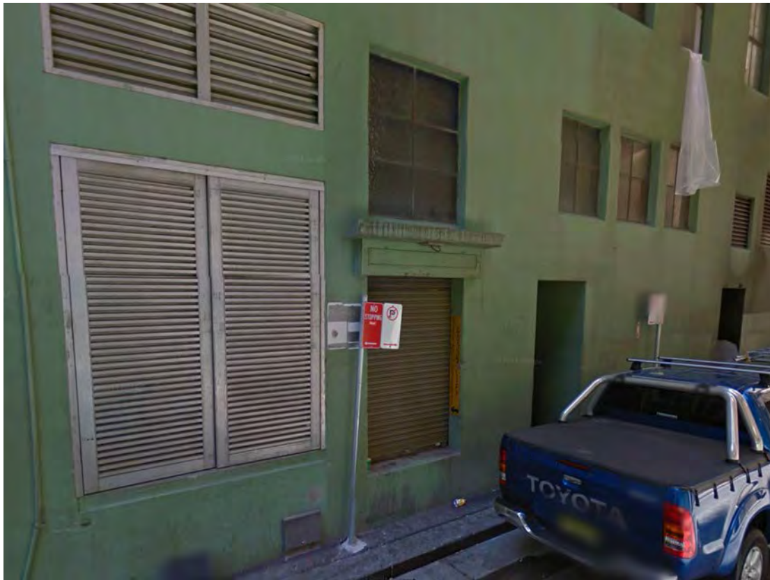
Figure 38 – View of external opening for York Street Foyer goods lift, from York Lane. At present, while the roller door is operable, the internal lift shaft has been closed off behind this opening with a masonry wall.
