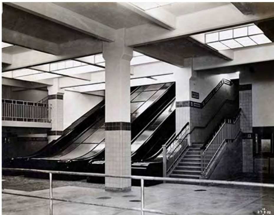
Figure 20 – The above scene of the Wynyard concourse in closer detail, showing the escalators up to the York Street entrance, taken 27.2.1932. The concrete floor finish is quite clear in this photo. Note also the fire stair to the proper left of the escalators, with original geometric pattern wall tiling. (Image source: State Records of NSW: Photo Investigator, ID #12685_a007_a00704_8735000031r ).
