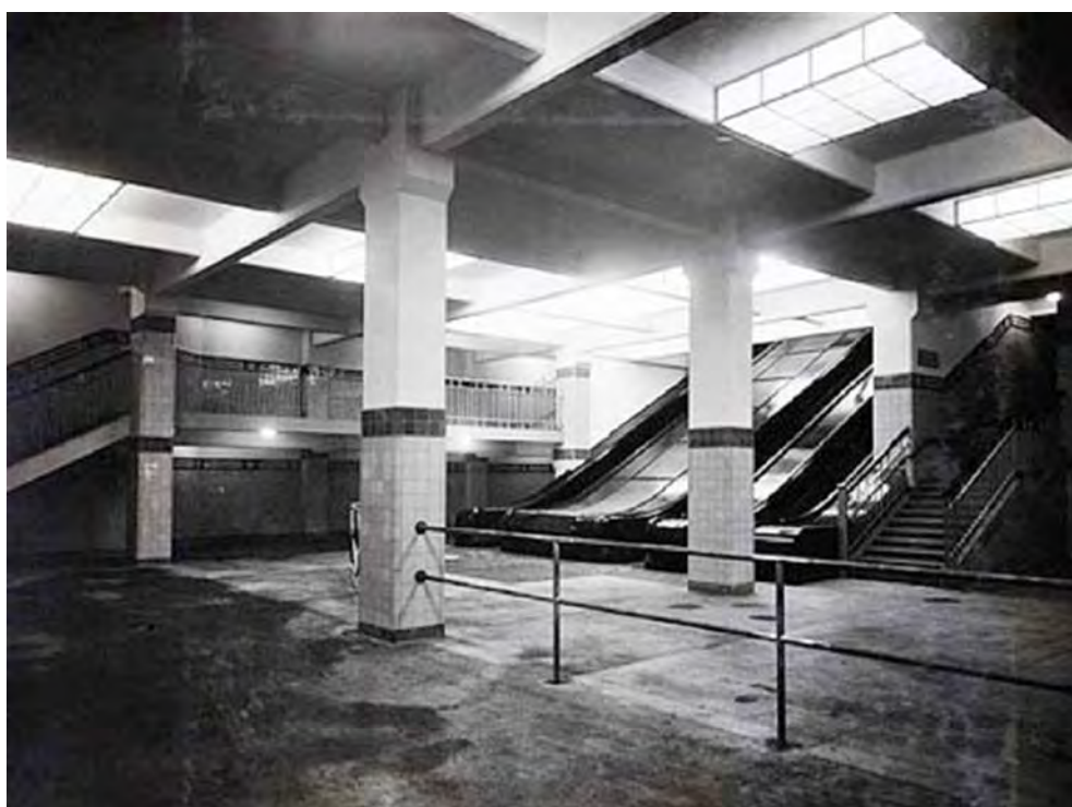
Figure 19 – Photograph of the Wynyard concourse, showing the escalators up to the York Street entrance, taken 27.2.1932. Note the box light fittings and the wall/column tiling configuration. Other original features visible in this photo include the Basement level 3 mezzanine level (background, left), the York Street fire stair
