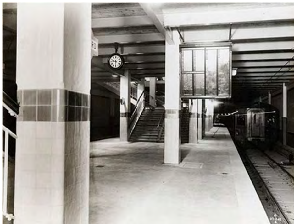
Figure 22 – Photograph of Platforms 5 & 6 (allocated for the City Circle services), taken 27.2.1932. The tiling on the columns can be seen to sit just below the chamfered detail (Image source: State Records of NSW: Photo Investigator, ID #12685_a007_a00704_8735000028r).
