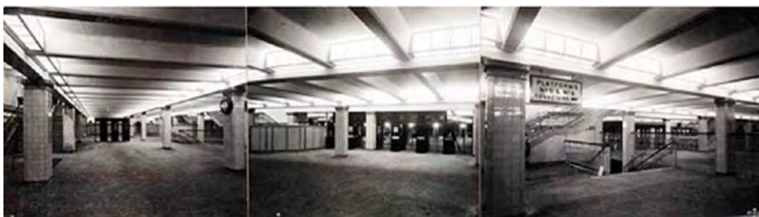
Figure 16 – A compiled panorama photograph of the Wynyard concourse, taken 27.2.1932, just prior to the opening of the Station. Note the box-shaped strip lights fitted into the ceiling throughout the station ( Image source: State Records of NSW: Photo Investigator, ID #12685_a007_a00704_8735000035r ).
