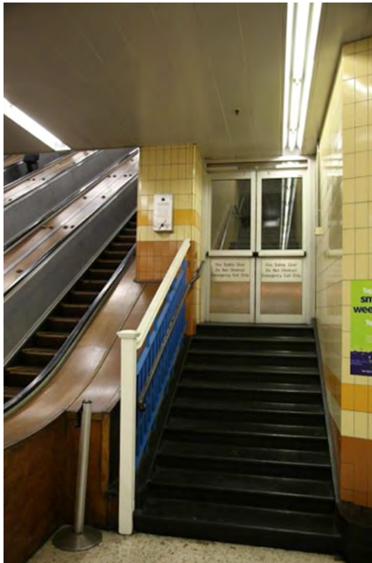
Figure 96 – The eastern fire stair within the western concourse. This stair is to be removed from B4 and B3 to commence at B2 (Image source: Futurepast 22/08/2014)
