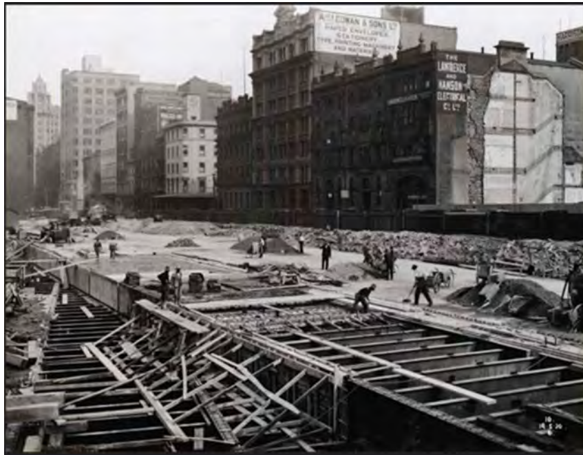
Figure 60 – Pouring the roof slab over Wynyard Station during its construction in the 1930s. Photograph dated 19 May 1930. (Source: State Records NSW, image ID 12685_a007_a00704_8735000019r.jpg)
