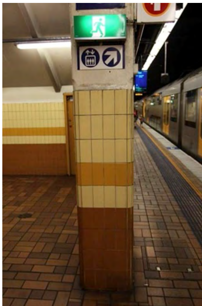
Figure 74 – Photograph of Platform 5, showing the non-original wall and column tiling which is to be replaced (Futurepast 2013).
