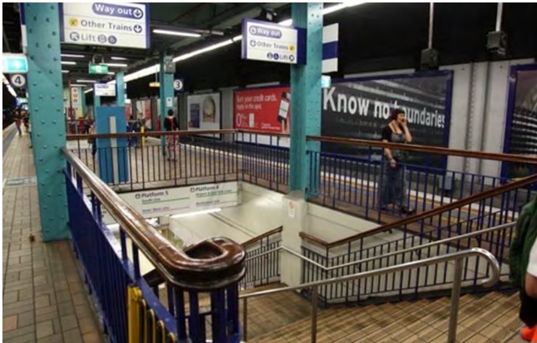
Figure 73 – View of Platforms 3 and 4. The original balustrading to the stairs and the riveted girder columns are to be repainted ( Futurepast 2013 ).
