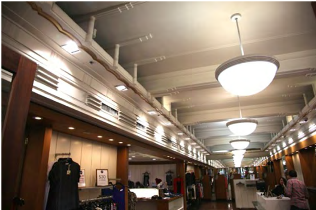
Figure 84 – Retail spaces in the northern unpaid concourse with areas of original ceiling, moulded fibrous plaster (Image source: Futurepast 22/08/2014)
