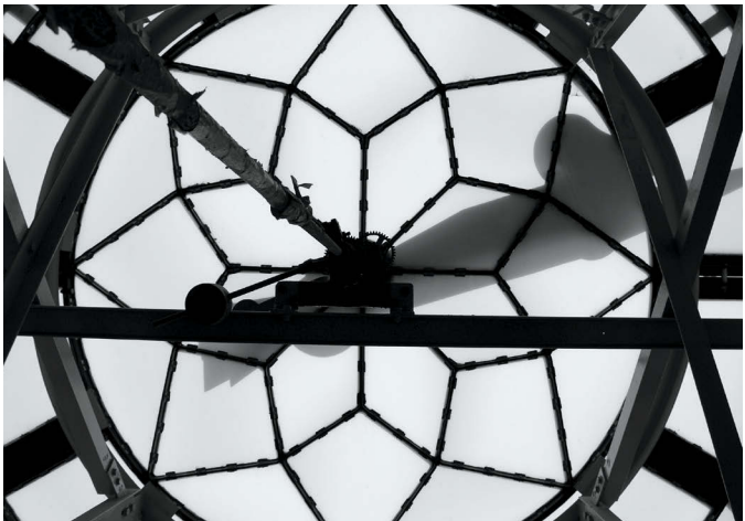
Figure 28: Looking through the glass of the Central tower clock face, showing the winding rod that was part of the original mechanism and is still used to turn the hands (Source: Sydney Trains)
