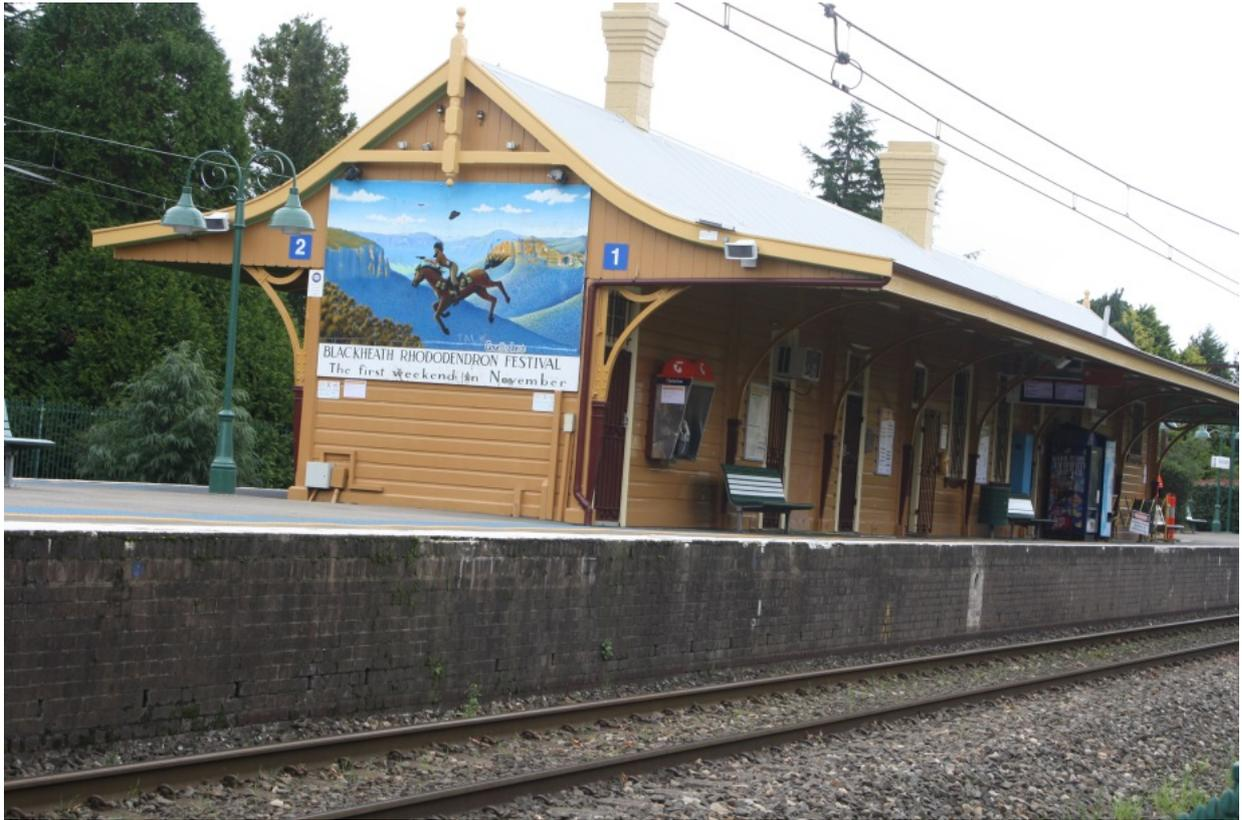
Figure 7 View north of 1898 section of platform 1 showing two courses of brick additions above the original
