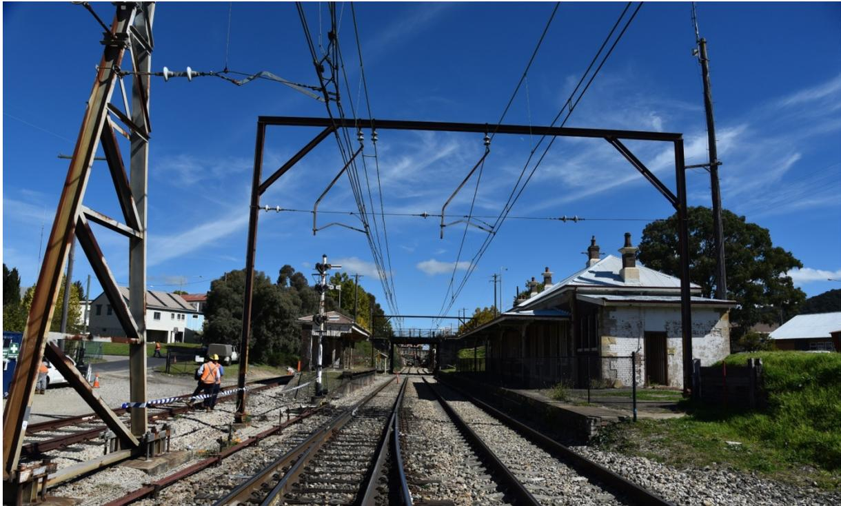
**Figure 8: Western main lines near station platforms, showing portal overhead wiring structure and signalling lights. West aspect**
