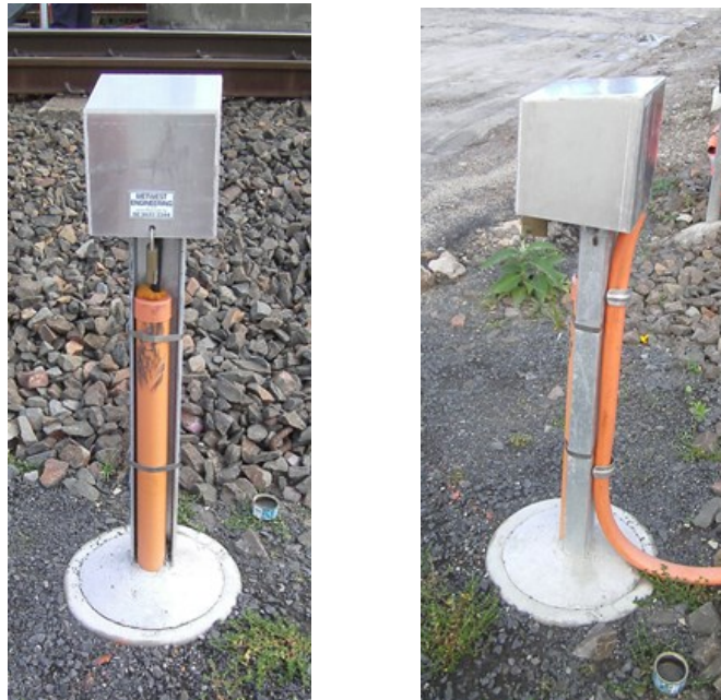
Figure 17 - Above Ground Balise Junction Box on a Standard Post.
