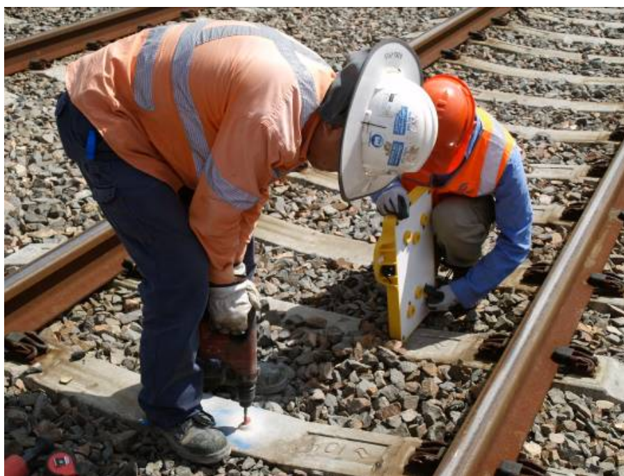
Figure 50 - Drilling of Concrete Sleeper In Preparation for Fitting of Anchors
