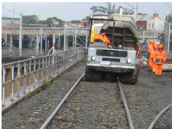
Figure 48 - A Wide Tyred Dump Truck on the Track
