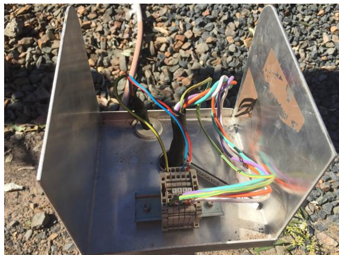
Figure 18 - Above Ground Balise Junction Box with Lid Removed.
