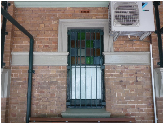
Figure 5-31. Detail of original 'cathedral glass' window panes, moulded render architraves, string course and window sills.
