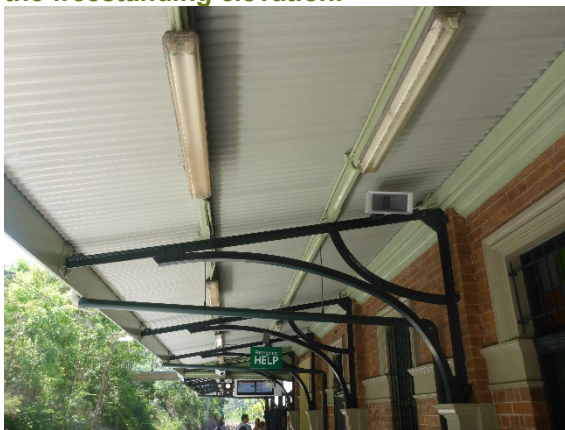
Figure 5-29. Detail of gabled roof and cantilevered curved cast iron brackets.
