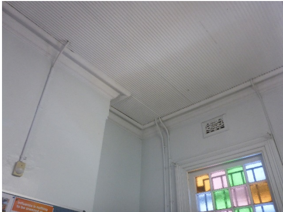
Figure 5-37. Detail of original corrugated iron ceiling panels and decorative cast-plaster air vents in the station masters office.
