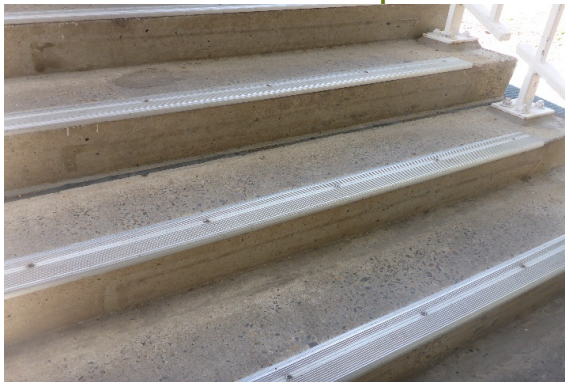
Figure 5-25. Detail of nosing on stairs.
