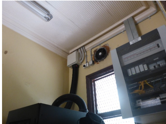
Figure 5-44. Interior of the store room (former booking office) showing an ETS primary enclosure for equipment and conduits leading into original corrugated iron ceiling.
