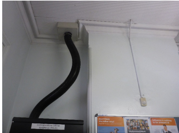
Figure 5-38. Detail of existing conduit leading from the main switchboard to the corrugated iron ceiling.
