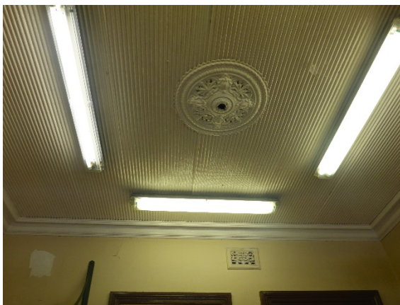
Figure 5-39: Detail of decorative mini orb ceiling fixtures which once accommodated a ceiling fan (now removed). Note unsympathetic addition of LED light fixtures.
