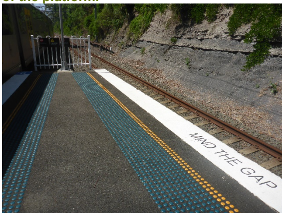
Figure 5-19. Detail of existing TGSIs along the station platform.
