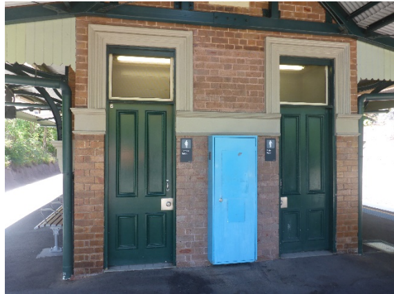
Figure 5-32. The northern elevation of the station building showing the entrance to the male and female bathrooms. Note the modified brick between each door where the wall was modified to accommodate each two entrance during upgrades to the station in 1995 and intrusive blue box secured to the wall.
