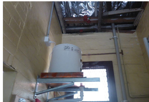
Figure 5-47. Detail of missing corrugated iron ceiling panels in the northern end of the storeroom (former waiting room).
