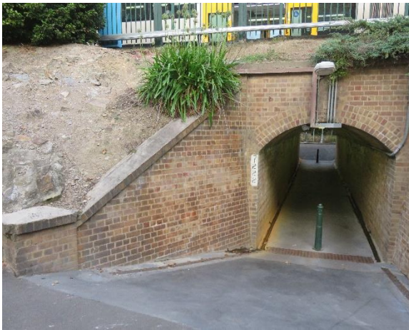
Figure 4.13 View west, showing brick abutments of underpass. (Source: GML)
