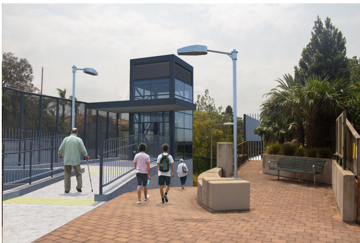
Figure 6.4 3D model showing the proposed new accessible pathway and lifts to Platform 1. (Source: Jacobs for Transport for NSW)
