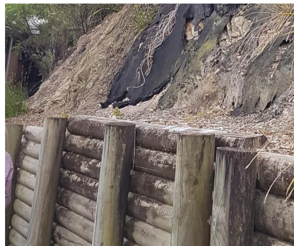
Figure 4.18 Log retaining walls. (Source: GML)
