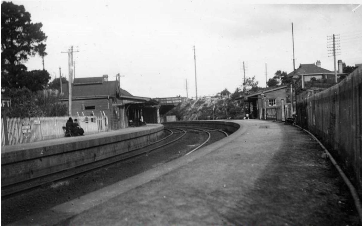
Figure 3.4 Photograph of Wollstonecraft Station looking from Platform 2 towards station buildings and platform 1, c1920s. Note platform is of brick construction and appears higher with a thickened brick edge. (Source: Australian Rail History Society)
