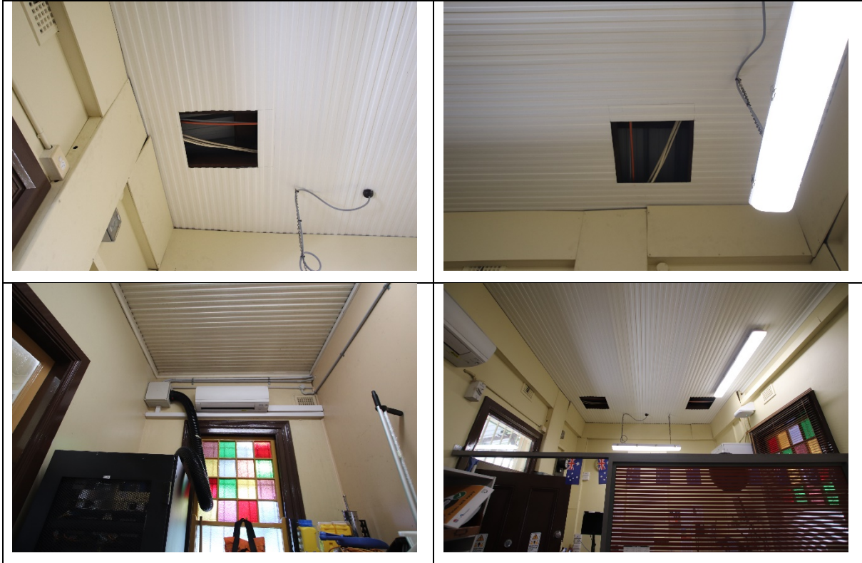
Plate 11 Views of the ceiling inside the station building. Penetrations were made recently to repair electrical faults in the ceiling
