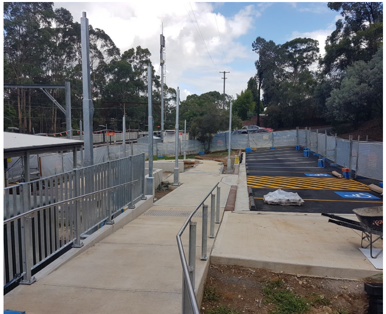
Above: construction progress in the lower commuter car park during February 2021.
