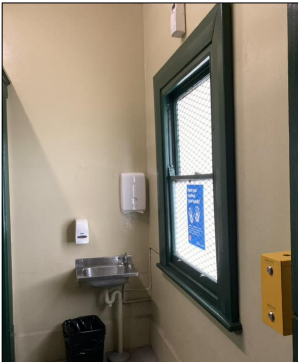
Photo 4.15 Female bathroom showing the original timber framed sash window
