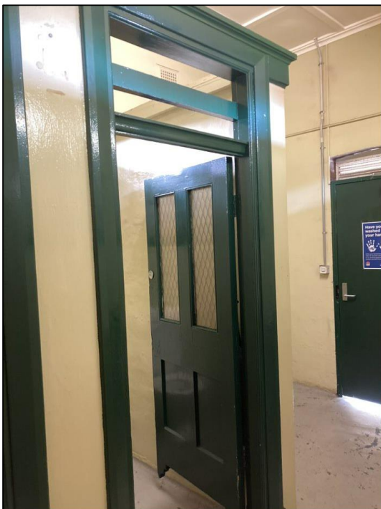
Photo 4.19 Original timber door retain glazing to the upper panels
