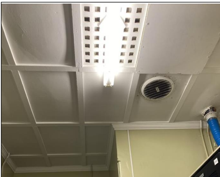
Photo 4.9 Timber batten and cement sheet ceiling with added lattice panel in station building
