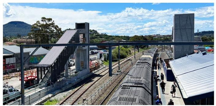
Scaffolding on the lift shaft on Berkeley Road West has been removed and the stair canopy installed.
