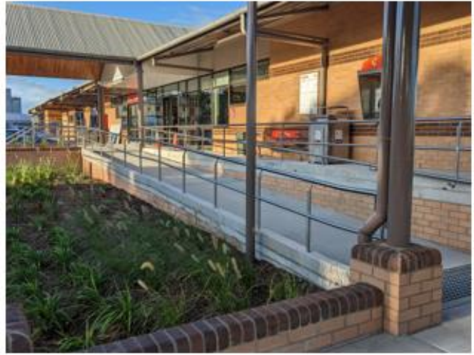
Access ramp at the front of the station
