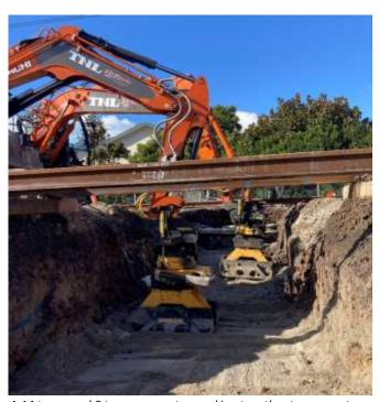
A 14 tonne and 8 tonne excavator working together to compact and stabilise the earth under existing tack, following the installation of an underline drainage crossing.
