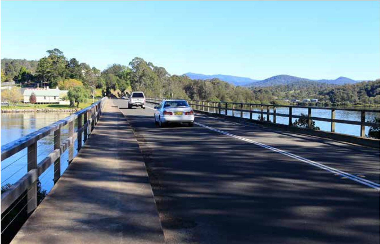
Photograph 2.11: Clyde River Bridge, Nelligen
