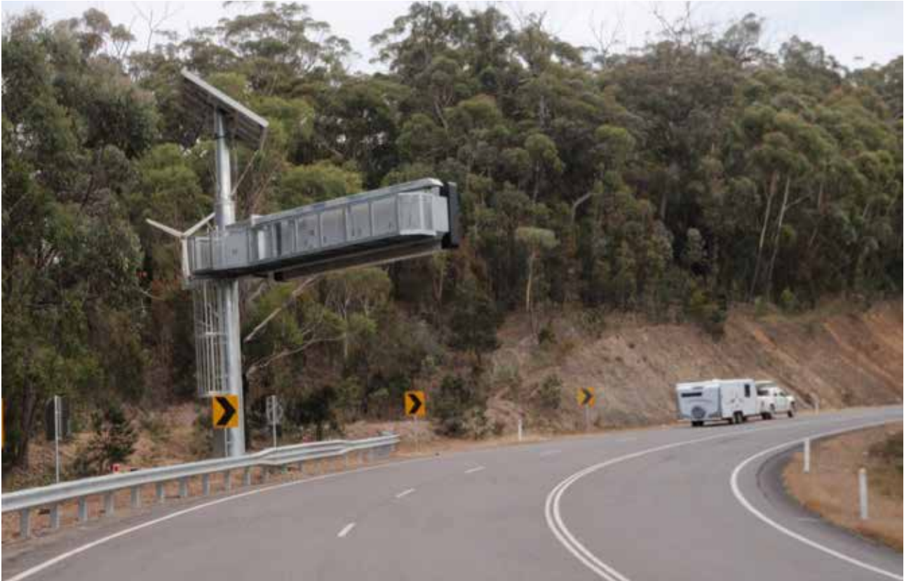
Photograph 2.13: Poorly located structure
