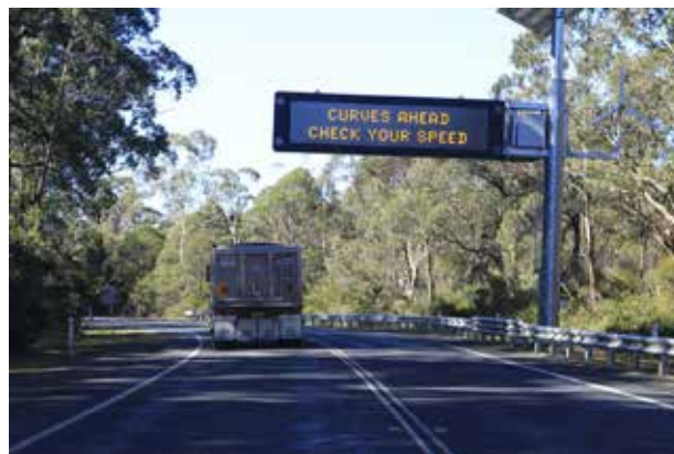
Photograph 3.6: Permanent VMS structure, eastern escarpment
