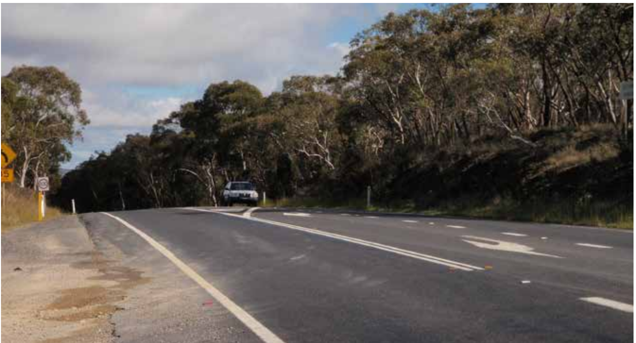
Photograph 2.2: Road junction on a crest
