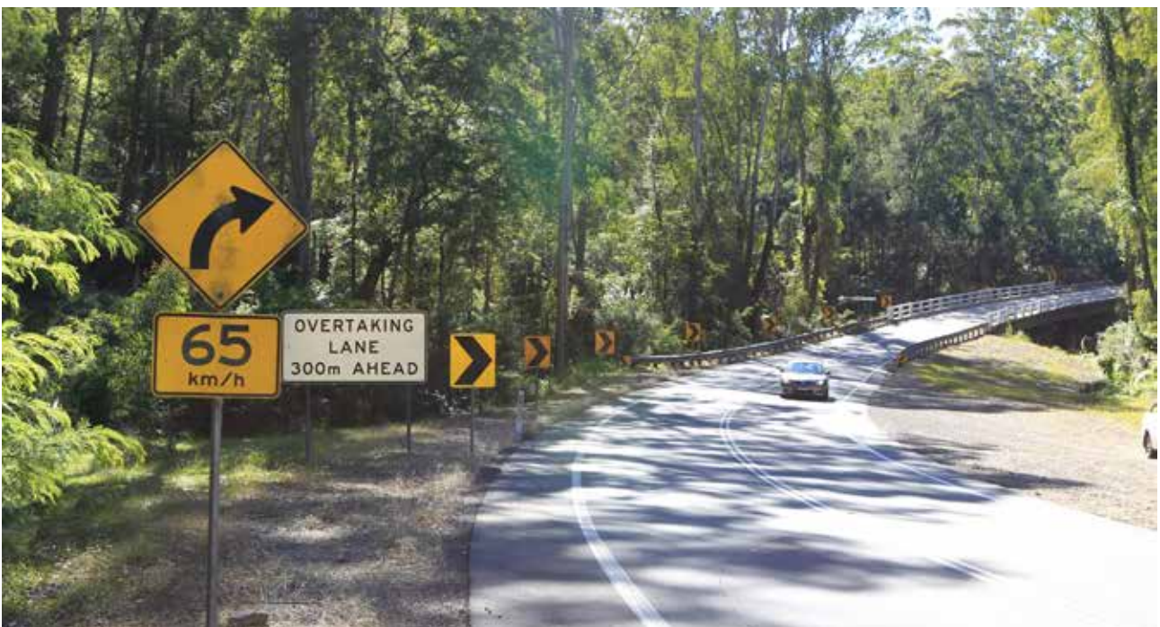
Photograph 1.5: Cabbage Tree Creek Bridge near Nelligen
