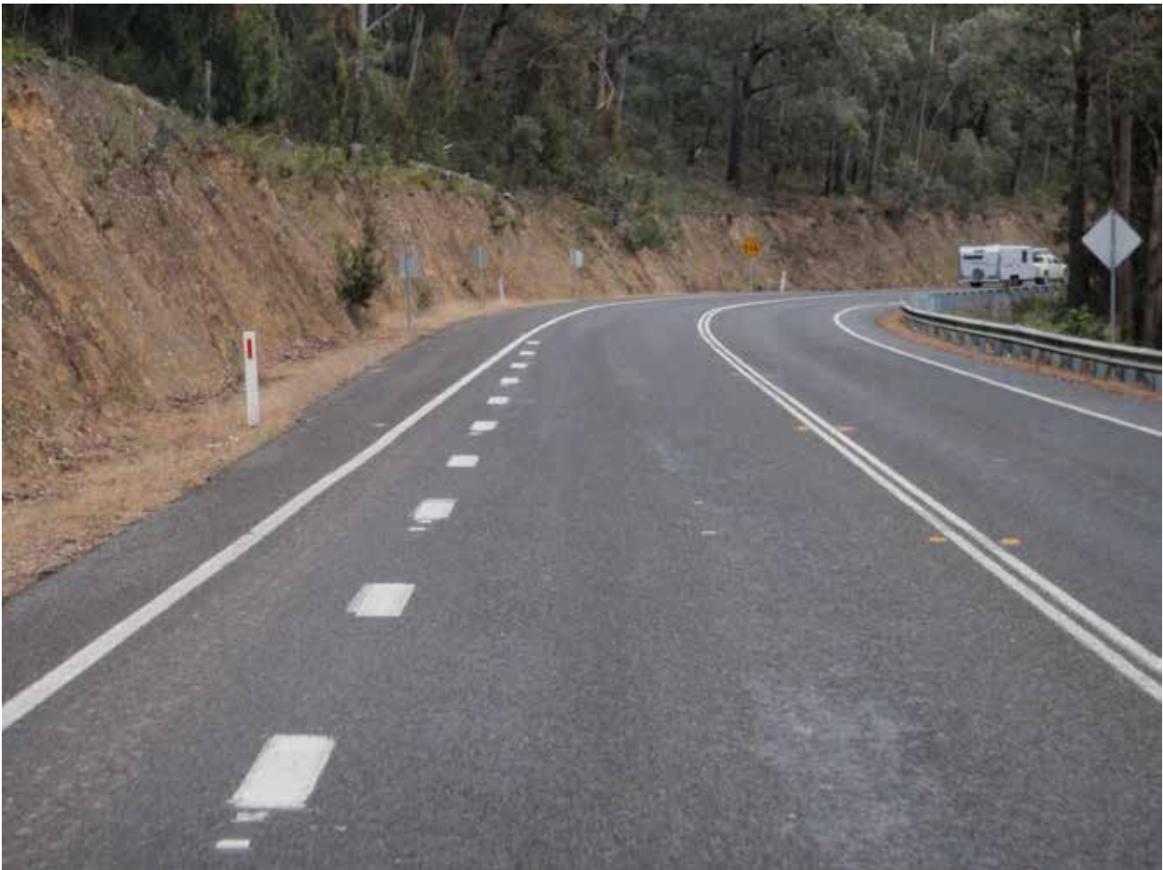
Photograph 2.8: End of an overtaking lane, Clyde Mountain
