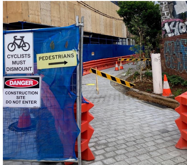
Photo 13 – Signage and traffic controls on Little Eveleigh Street. Bicycle parking in service, street paving complete and boundary fencing in place around LES Building works.
