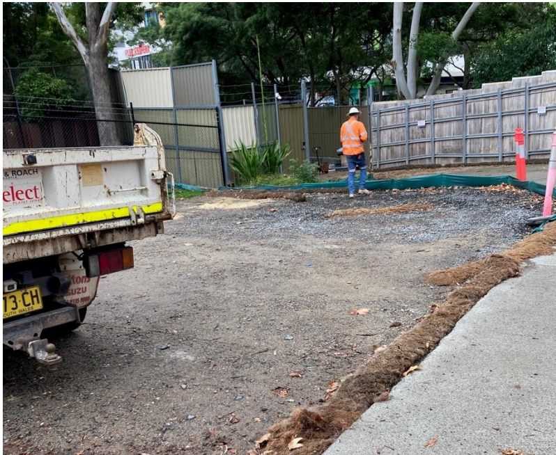
Photo 8 – Erosion and Sediment Controls installed in the Marian Street Compound.
