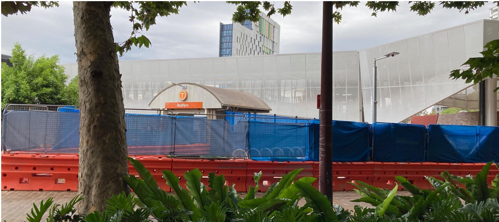
Photo 12 – Jersey and ATF fence barriers on Marian Street compound, and view of the new concourse behind.
