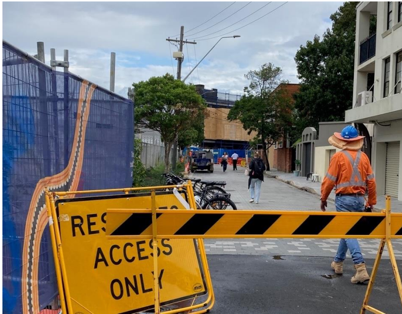
Photo 13 – Signage and traffic controls on Little Eveleigh Street. Bicycle parking in service, street paving complete and boundary fencing in place around LES Building works.
