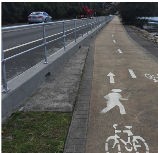
Brisbane Water Drive, Tascott – Hunter Region, May 2017. Safety project to install low level concrete barrier and handrail between road and shared use path.
