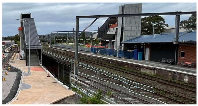
Coloured concrete footpaths have been poured and new lighting has started being installed on Berkeley Road West.
