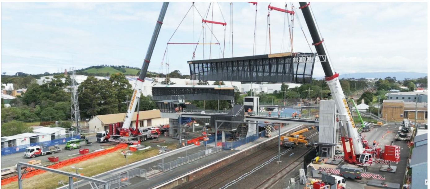
Canopies being installed on the new footbridge
