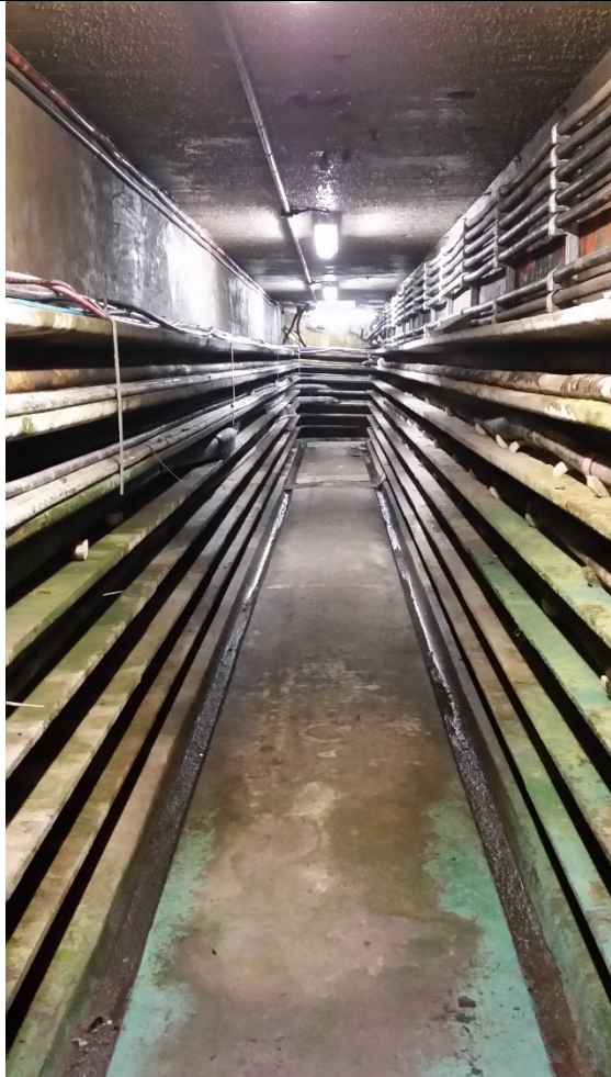
Plate 1 Service pit and tunnel
