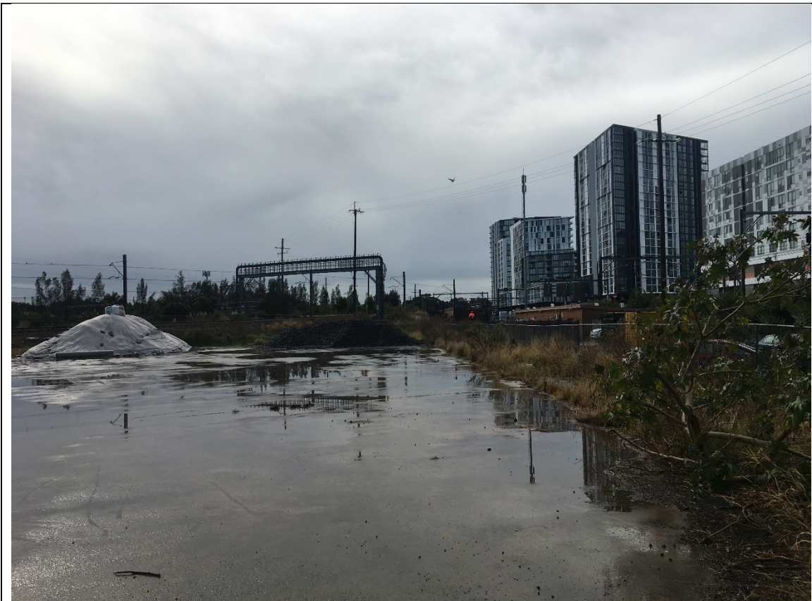
Plate 5 Wolli Creek Sectioning Hut and yard area to the south west of Wolli Creek Railway Station (sectioning hut proposed for demolition, yard to be excavated and used as a construction compound)
