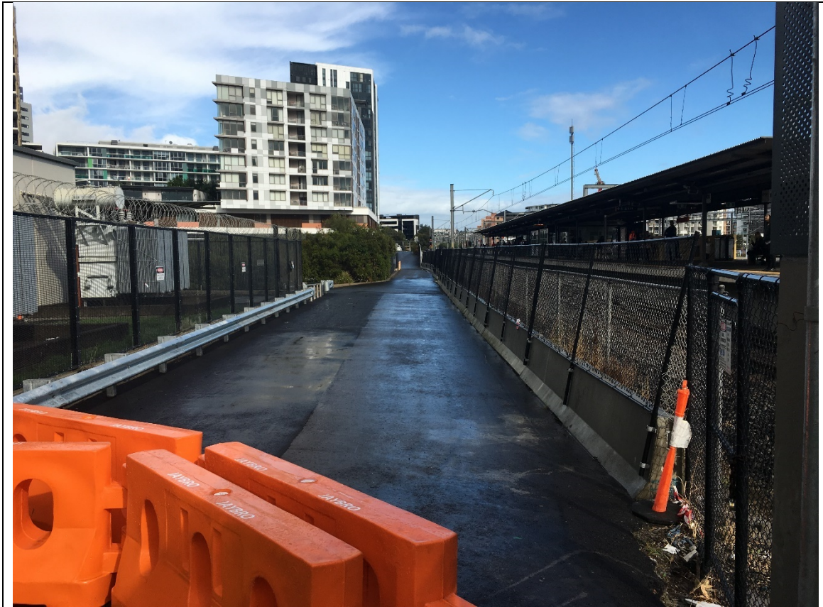
Plate 7 Undercliffe Substation (left) and Wolli Creek Railway Station (right) divided by Spark Lane
