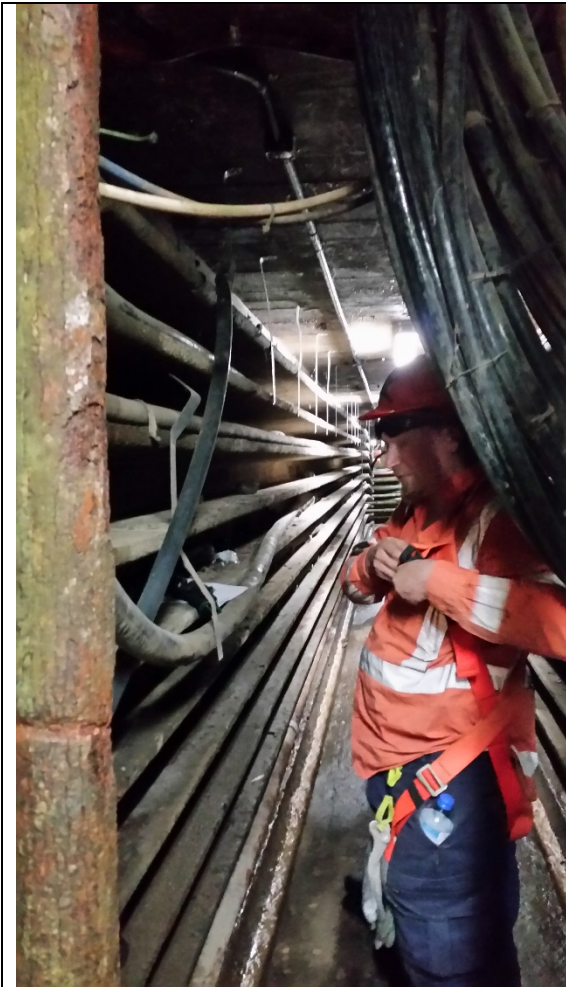
Plate 3 Service pit and tunnel with existing cables
