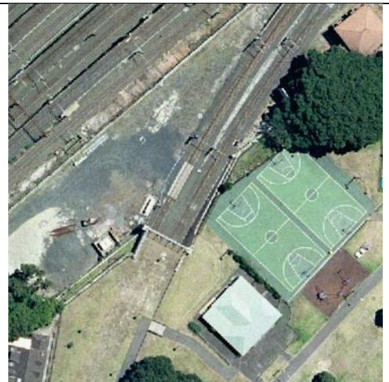
Figure 10 2000s aerial of the area proposed for trenching (after Airport tunnel works)
