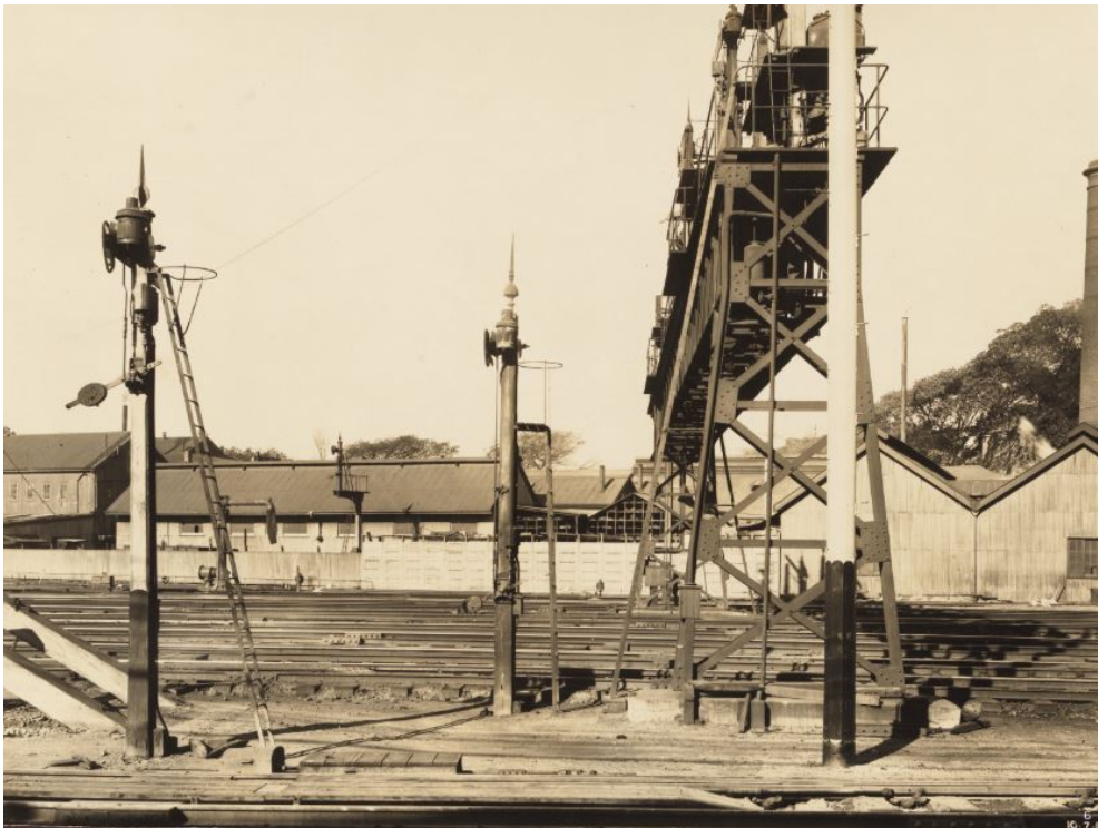
Figure 16 The chimney can be seen to the right, the now demolished structures to the left, circa 1915-1922 (Bradfield, 1922)
