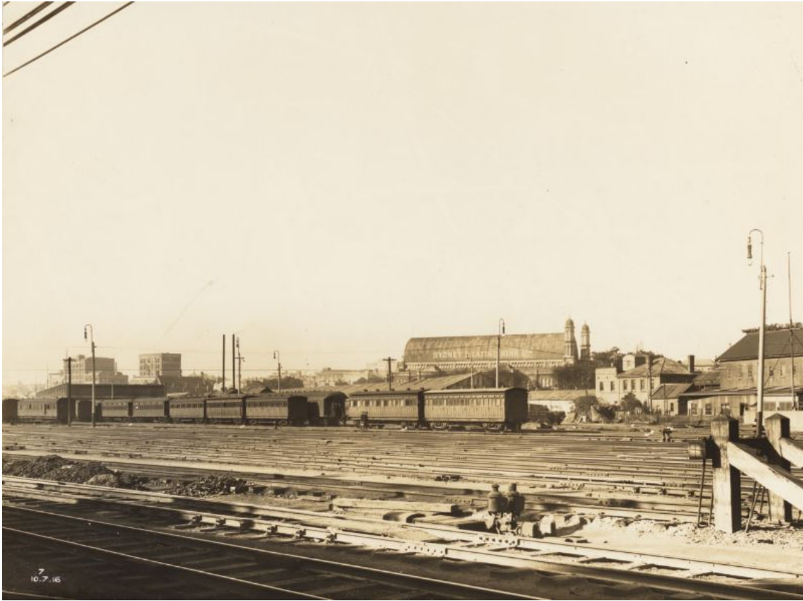
Figure 17 The former district engineers building and former draftsman's office, circa 1915-1922 (Bradfield, 1922)
