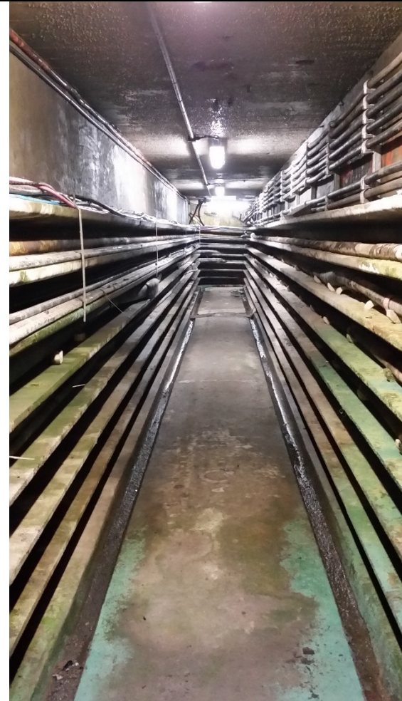
Plate 1 Service pit and tunnel
