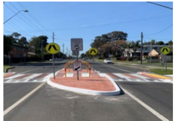
Raised pedestrian crossing on Cumberland Road Ingleburn at Ingleburn Public School, after completed works.
