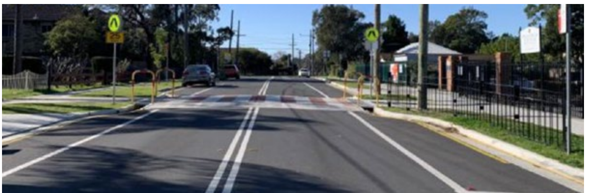
Raised pedestrian crossing at Ferndale Street, Revesby, after completed works.
