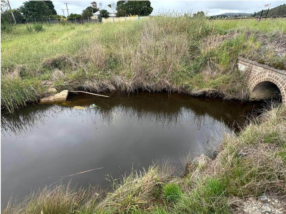
Photo 5: Downgradient of middle culvert with pooled surface water. Surface water was dark red/brown with minor turbidity.
