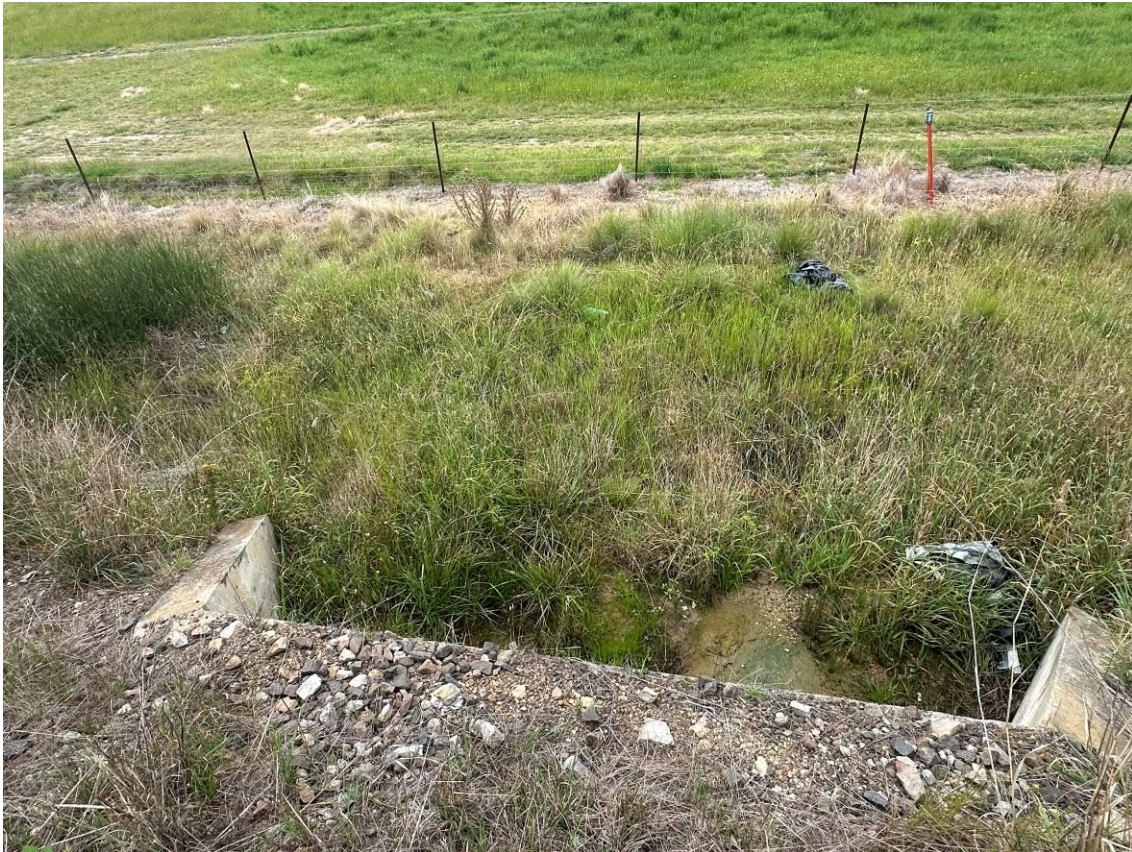
Photo 7: Downgradient of northernmost culvert with no surface water flowing off site. Soil was damp but no sediment build up was noted on nearby vegetation.
