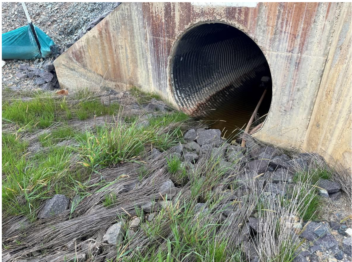
Photo 12: Upgradient of middle culvert with slow flowing/pooled surface water. Surface water was clear with a dark red/brown tint and with no to low turbidity.
