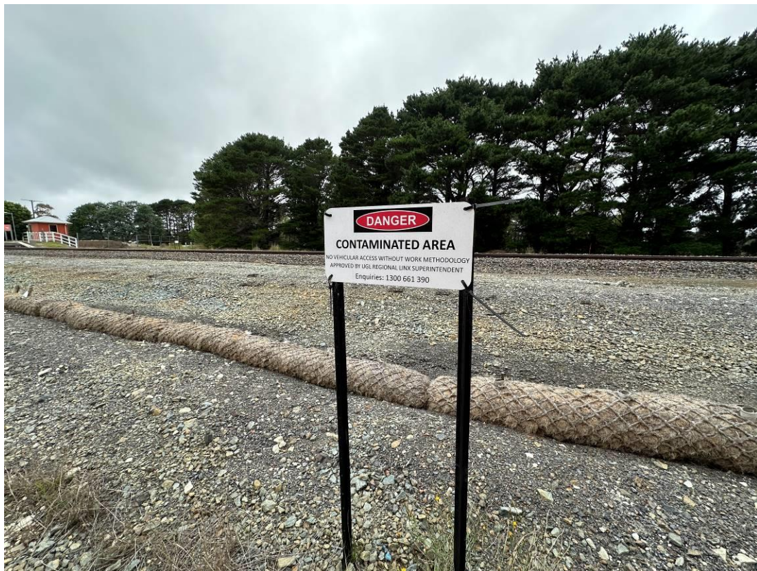
Photo 18: Contaminated land signage in good conditions, placed at appropriate intervals along the site.
