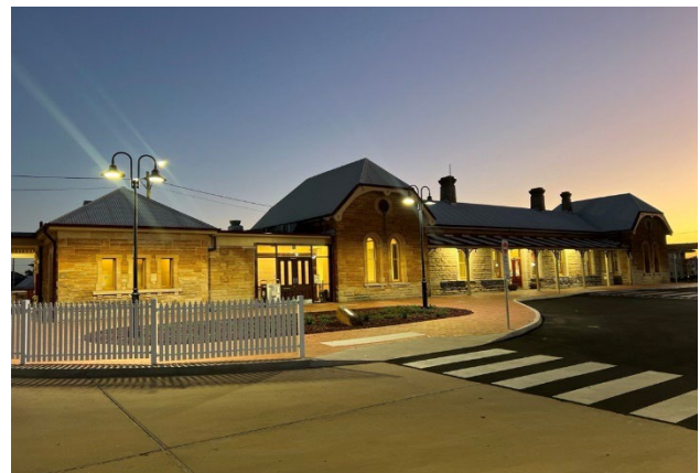
Above: Completed upgrade of Dubbo Railway Station including heritage light poles and improved wayfinding.
