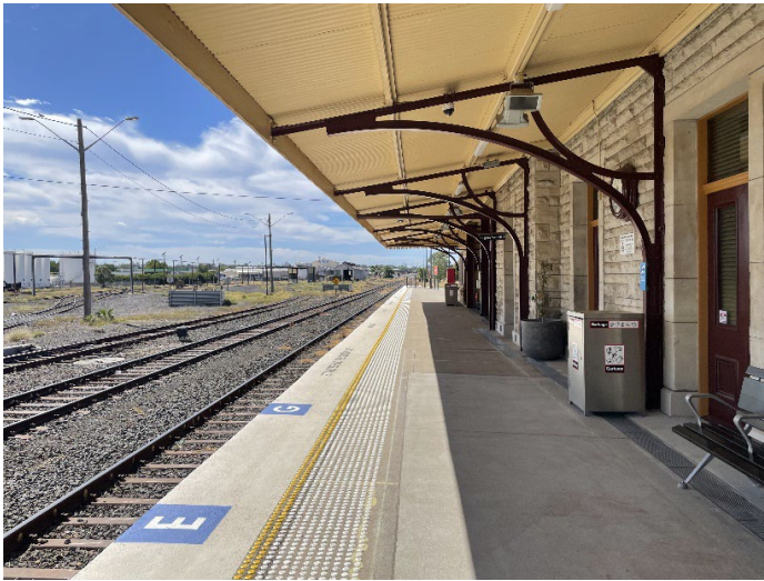
Above: Upgraded Station platform including regraded pavement, new drainage, and tactile indicators.
