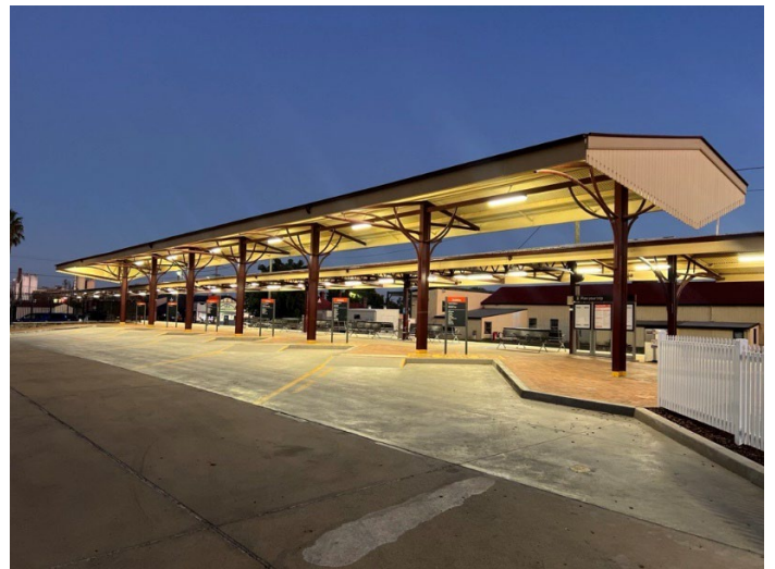
Above: Upgraded bus and coach bays with improved lighting and regraded pavement.
