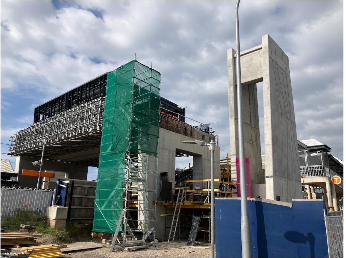
Stair and landing construction works on Platform 2.
