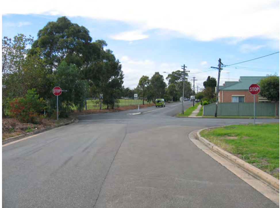
Figure 4 Looking east towards the intersection of Manchester Road and Chisholm Road
