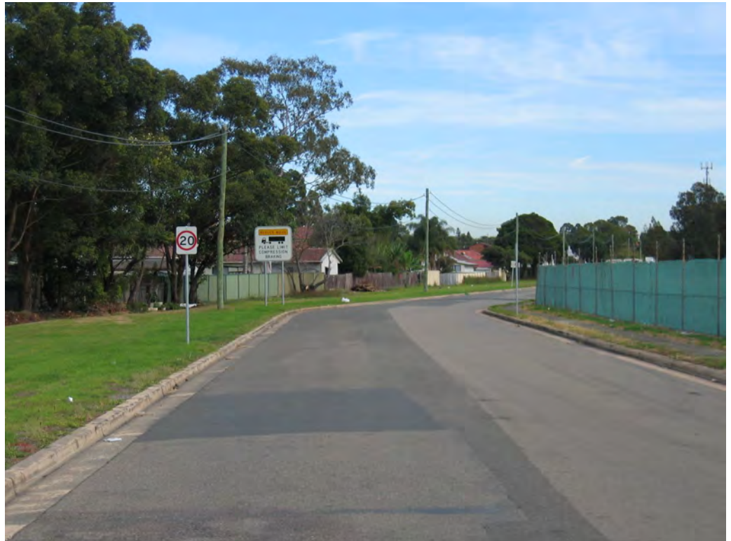
Figure 3 Looking west along the Private Road, located to the west of Manchester Road
