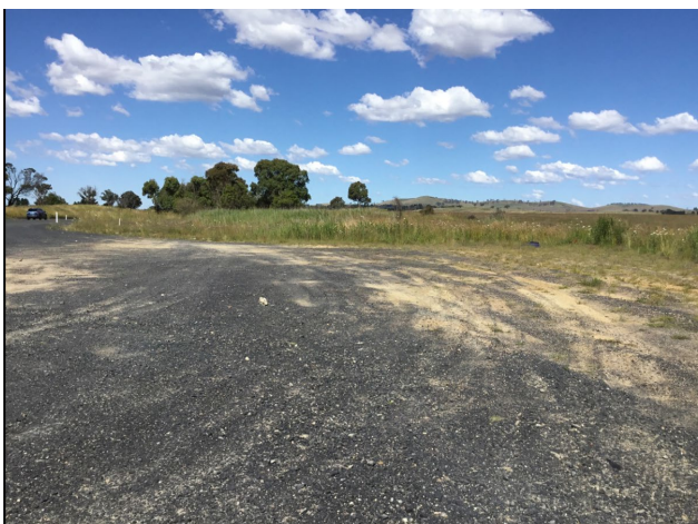
Figure 2-1 View north-east of existing spoil site and proposed compound site at Segment 1720/1725 southbound
