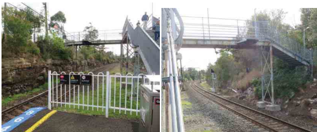
Figure 4-59: a) LEFT: Down Main - Facing Country from platform - OHW Attached to existing bridge, b) RIGHT: Up Main - Facing country from platform - OHW attached to existing bridge
