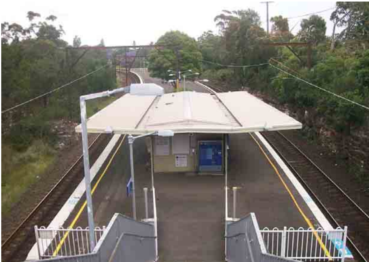
Figure 2-6 Existing structure at Mount Colah Station (facing south towards City)
