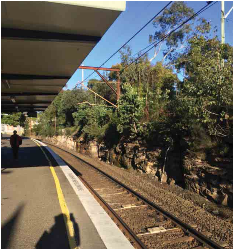
Figure 5-6 Vegetation along the western side (Down Main side) embankment
