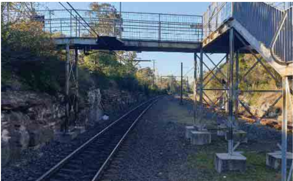
Figure 2-4 View of existing footbridge from platform (Down Main, facing north towards Country)
