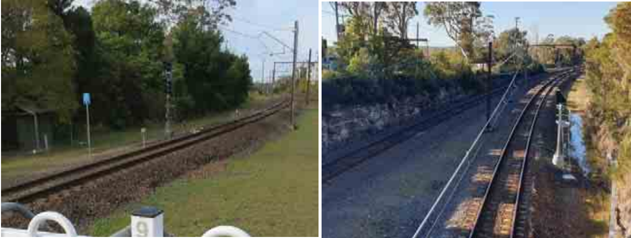
Figure 2-13: a) LEFT: Signal N23.48 at 37.568 km (View of Up Main towards city from Mount Colah Platform); b) RIGHT: Repeater N23.48 Signal at 37.774 km (View towards country from existing footbridge)
