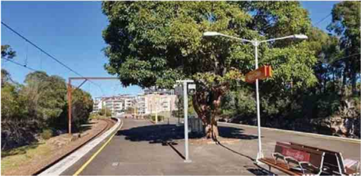
Figure 5-7 Shade tree - south end of platform (facing south towards Sydney)
