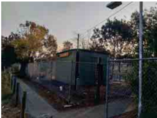
Figure 6 Mt Colah Station Signal Loc N23.48R
