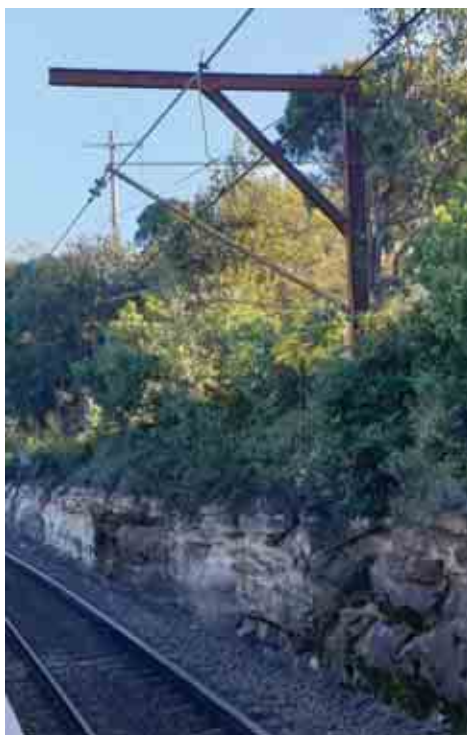
Figure 4-61: Existing OHWS N37+722
