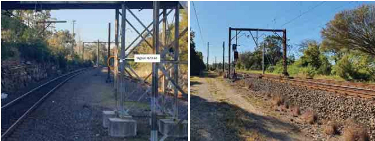
Figure 2-14: Signal N23.61 at 37.996 km a) LEFT: View of signal from Northern end of Mount Colah Platform, b) RIGHT: View towards country from Down access track
