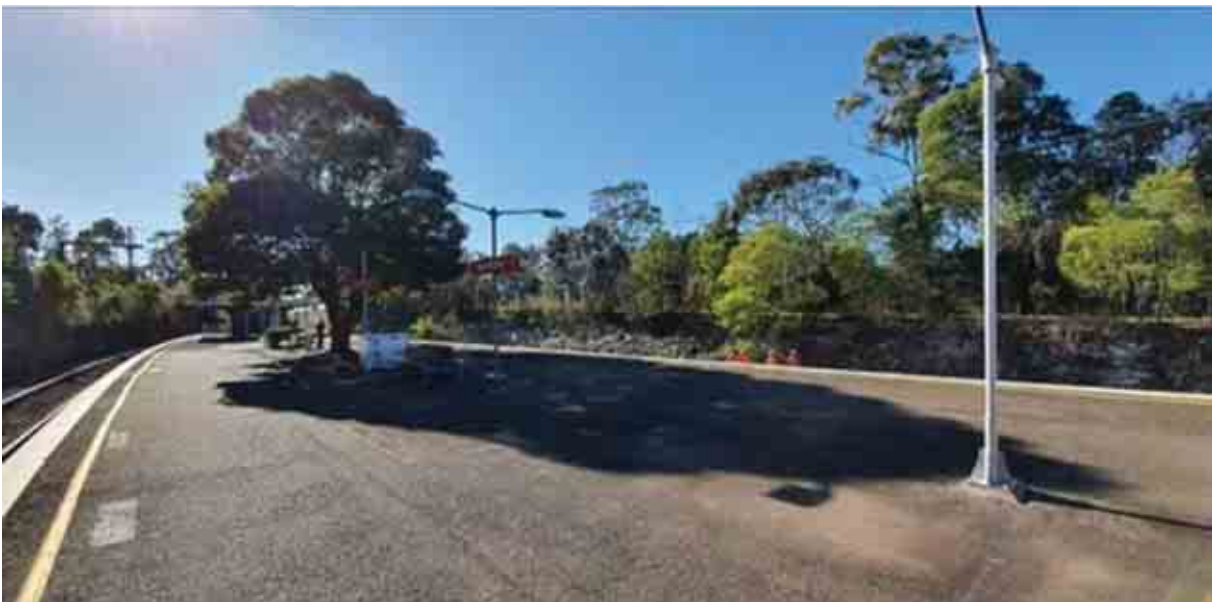
Figure 5-8 Shade tree - south end of platform (facing north towards existing footbridge)
