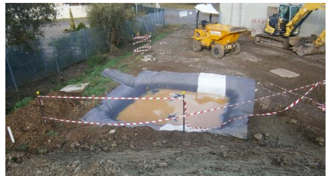
Figure 2: Sediment trap implemented to capture course sediment in confined spaces. Source: M5WW Project.
