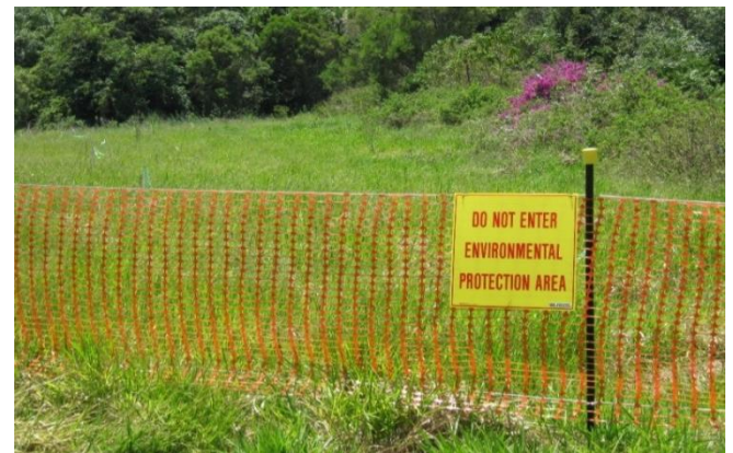
Figure 16: Para-web and signage installed on-site to identify and protect retained vegetation for unintentional impact.
