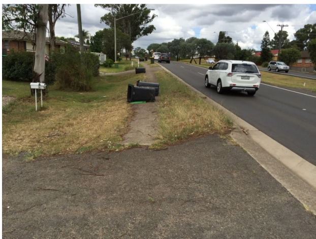
Current resident property access arrangement onto TNR – east side of TNR, Jamison Road to Smith Street
