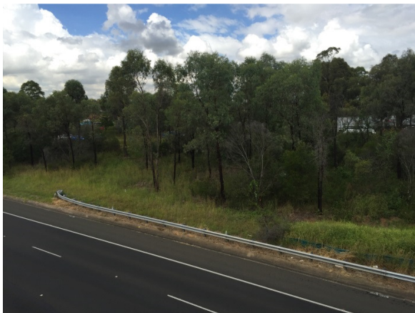
Clearing required at the southern abutment to facilitate the new bridge alignment.
