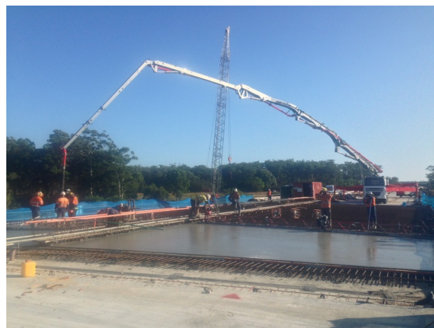
Pacific Hwy Upgrade – Oxley Hwy to Kundabung: pouring a 22m wide bridge deck.
