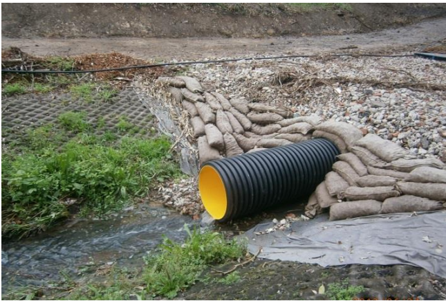
Figure 5: Temporary diversion pipe installed to facilitate access over drainage lines while still maintaining clean water drain. Source: M5WW Project.
