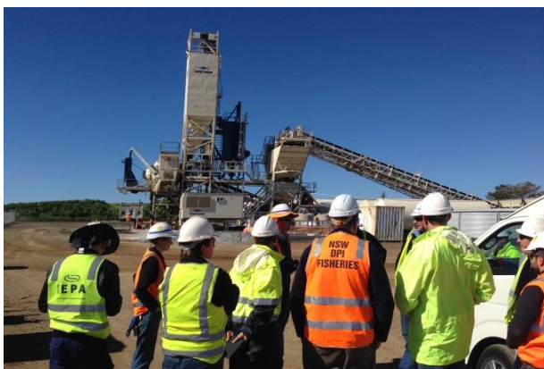
Figure 9: ERG group undertaking a guided inspection of the project at T2E.
