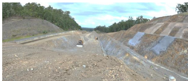
Lendlease excavating a large cutting. Source: Oxley Highway to Kundabung Project.
