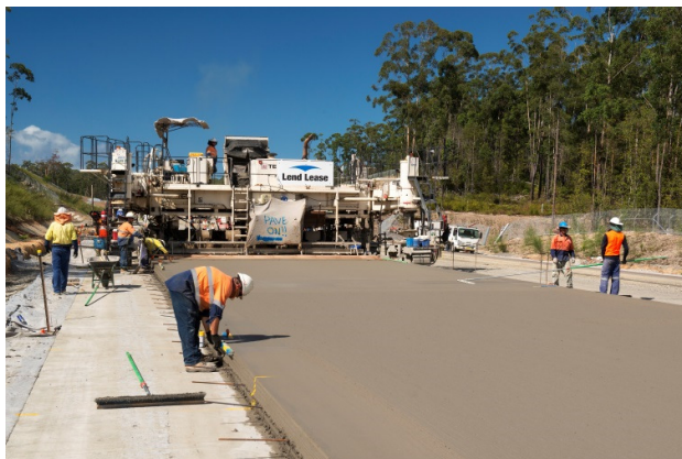
Nambucca to Urunga Pacific Highway Upgrade – Concrete Paving.
