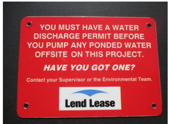
Figure 20: Notification tags installed on all pumps at T2E to remind personnel about the requirement to have an approved environmental discharge permit prior to dewatering.
