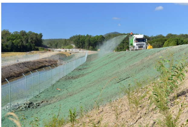
Nambucca to Urunga Pacific Highway Upgrade – Batter Protection
