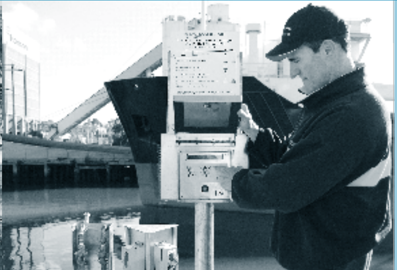
Environmental Service Officer, Paul Skimmings, gathers usage data from a vessel pump-out facility.
