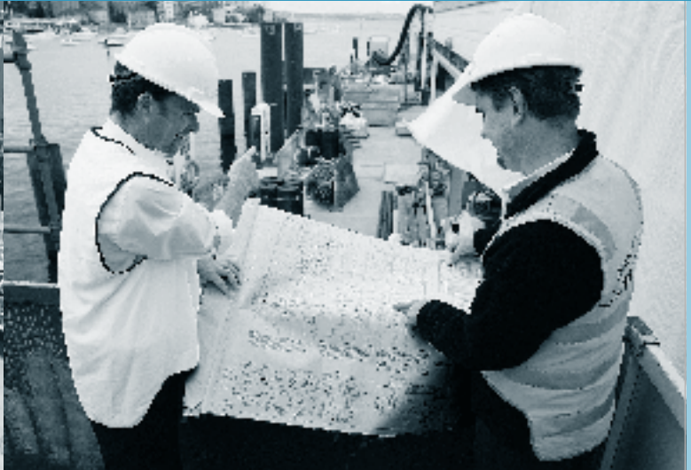
NSW Maritime's Principal Engineer, Patrick McCallum (at left), and contract Project Manager, Greg Westwood, discuss progress of the $15.7 million upgrade to Manly Wharf.
