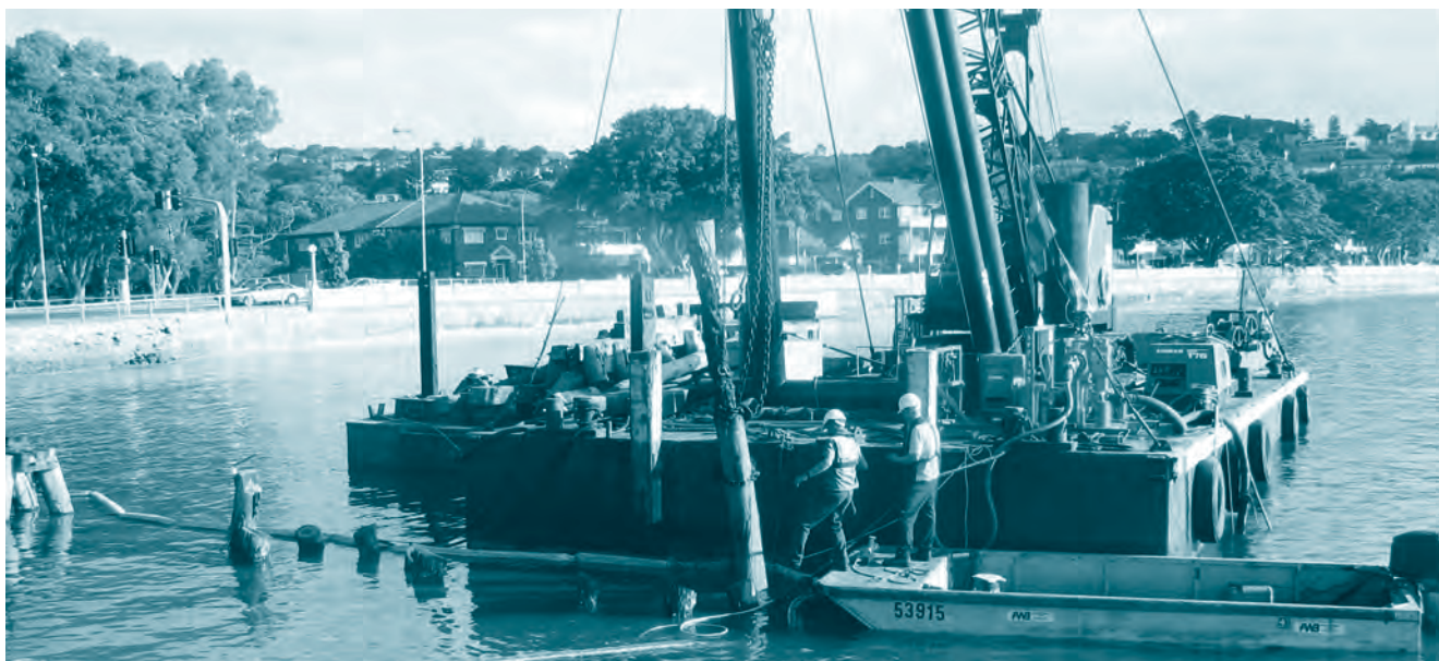
The old and disused former floating restaurant at Rose Bay was removed during the year along with associated navigational obstructions such as timber piles that had been driven into the bed of the harbour.
