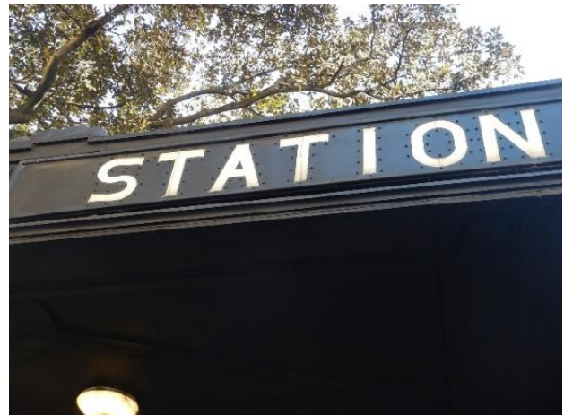
Figure 22: Original station signage on copper fascia cladding
