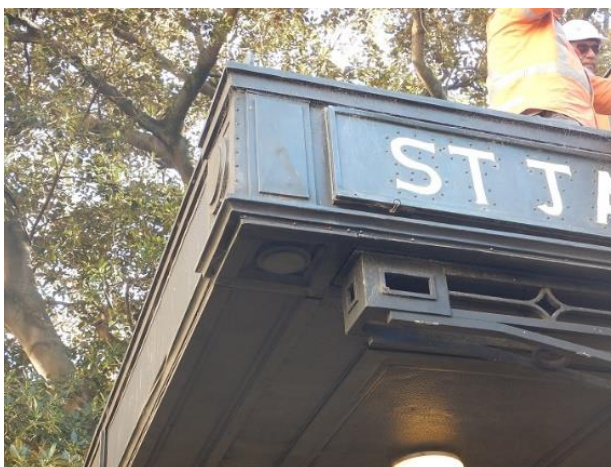
Figure 23: South west corner of awning fascia
