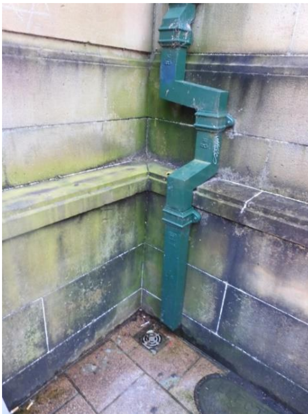
Figure 13: Cast iron downpipe on southern façade of entry building
