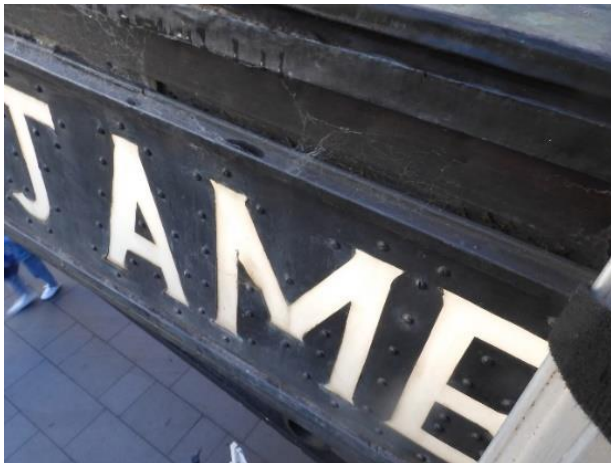
Figure 21: Original station signage on copper fascia cladding
