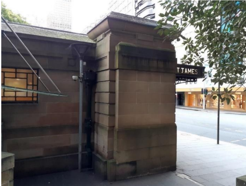
Figure 15: Cast iron downpipe on northern façade of building
