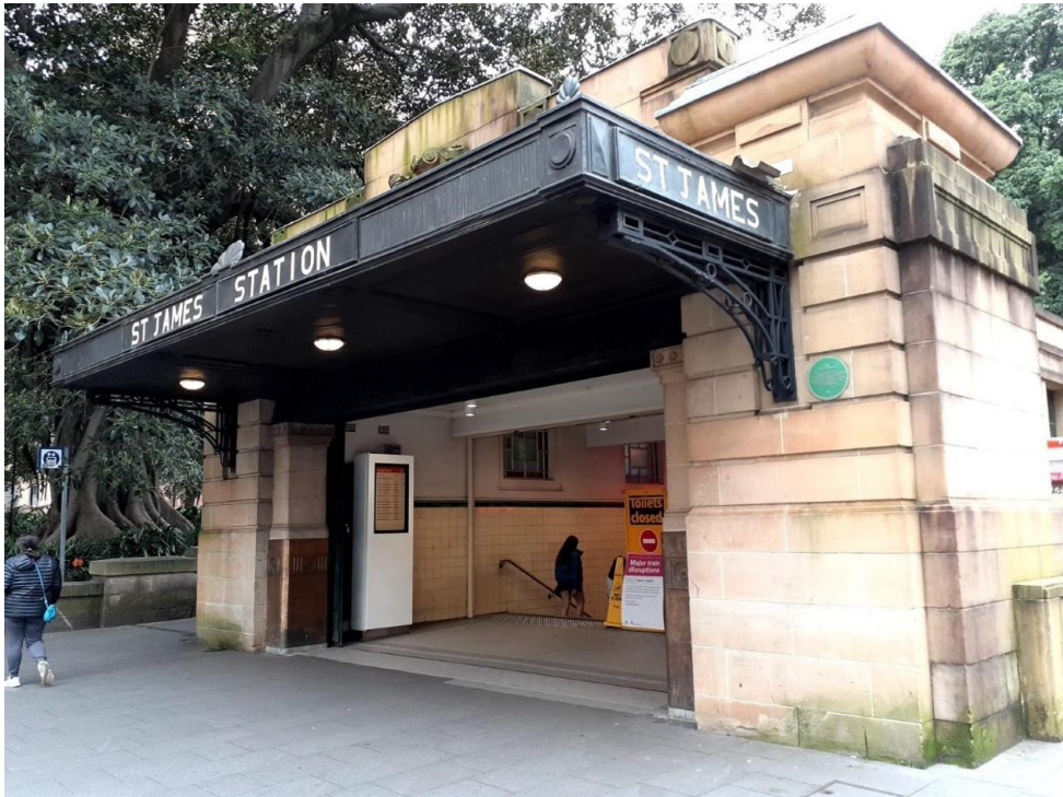
Figure 8: Elizabeth Street entrance awning looking north east.
