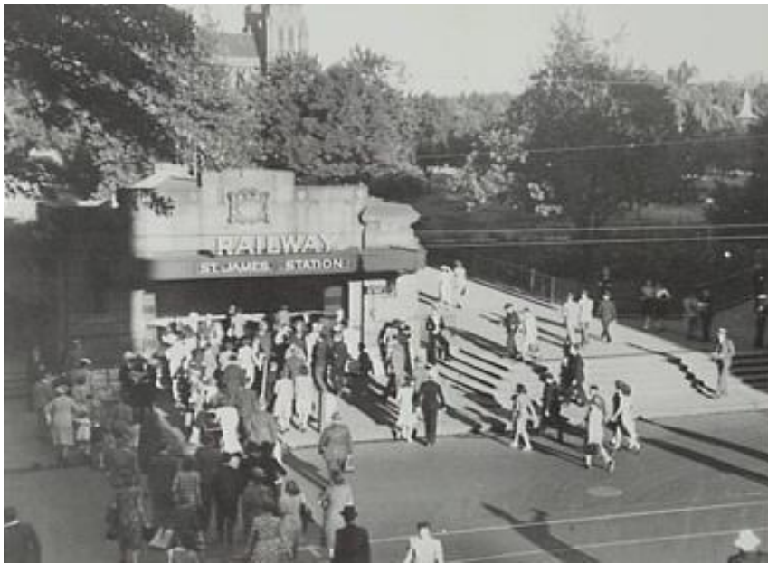
Figure 4: St. James Station (looking east) c. 1940. (Source: City of Sydney Archives)
