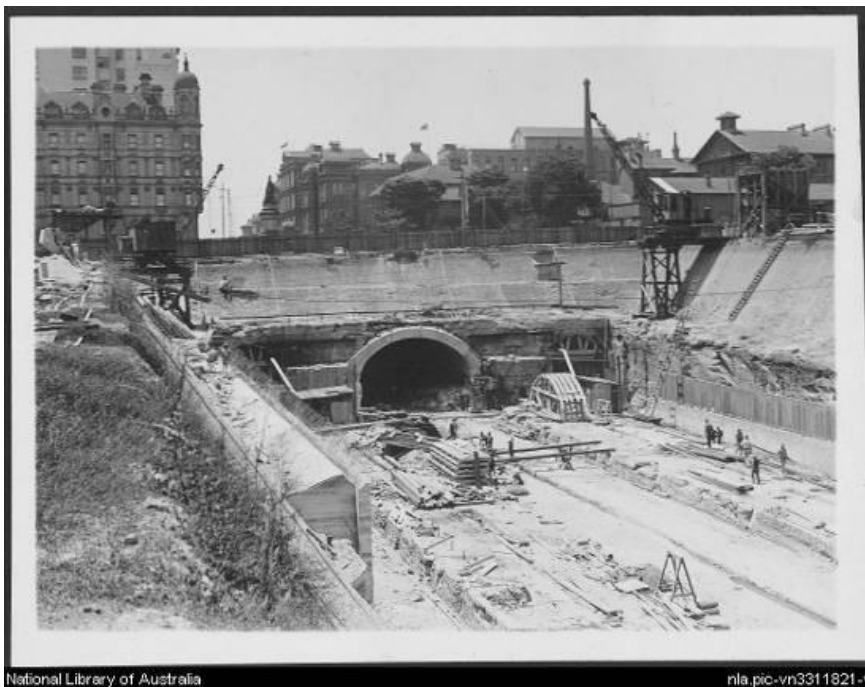
Figure 3: Construction of St. James Station (looking north) c.1925. (Source: National Library)
