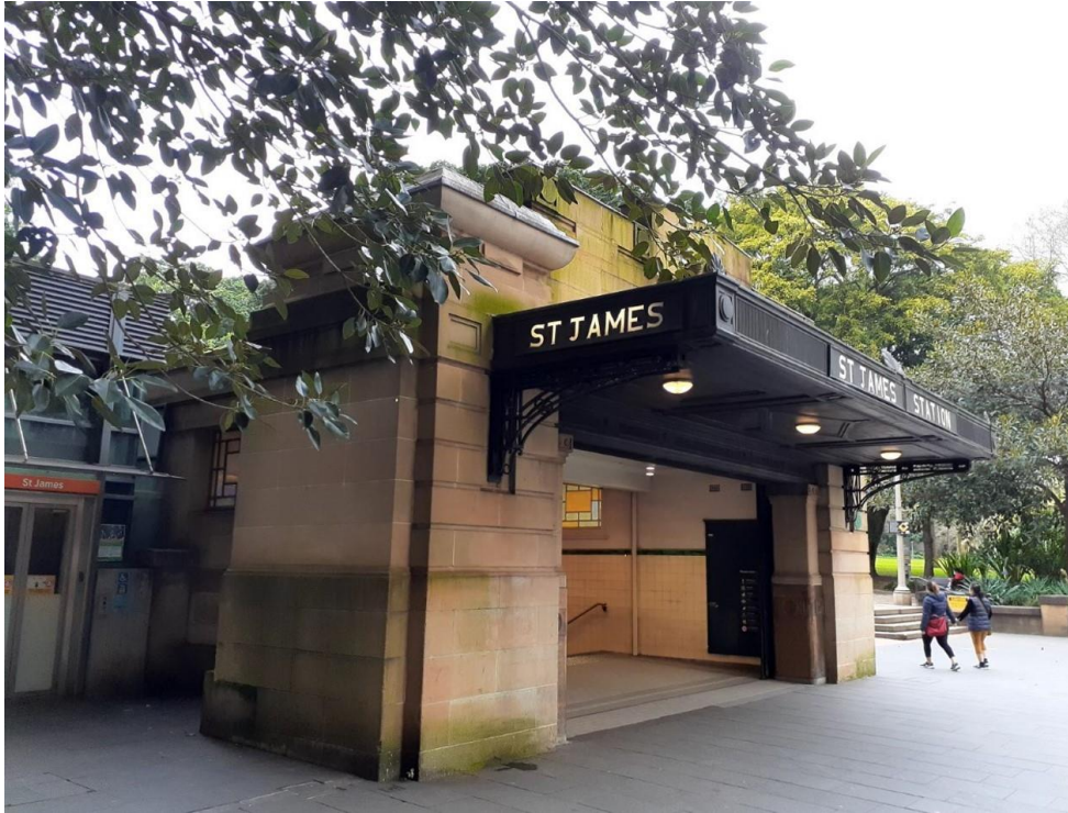
Figure 9: Elizabeth Street entrance awning looking south east.
