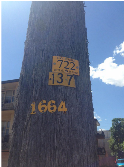
Photo 2. Sydney Trains OHW power pole identification
