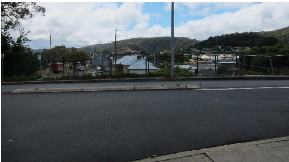
Figure 28. View east from the Bridge Street Overbridge toward the roofscapes of the Eskbank Railway Station group. (Source: Heritage Now 2023)
