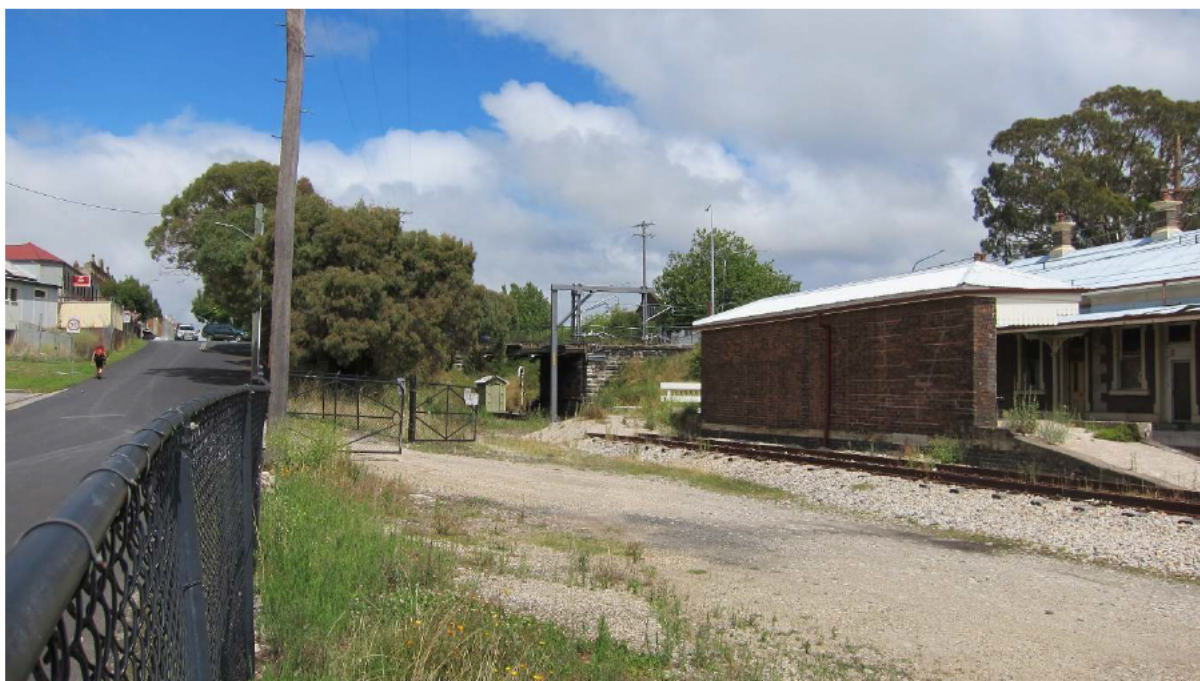
Figure 26. View north west from Gas Works Lane across the Eskbank Railway Station group toward the sandstone abutments of the Bridge Street Overbridge. (Source: Heritage Now 2023)
