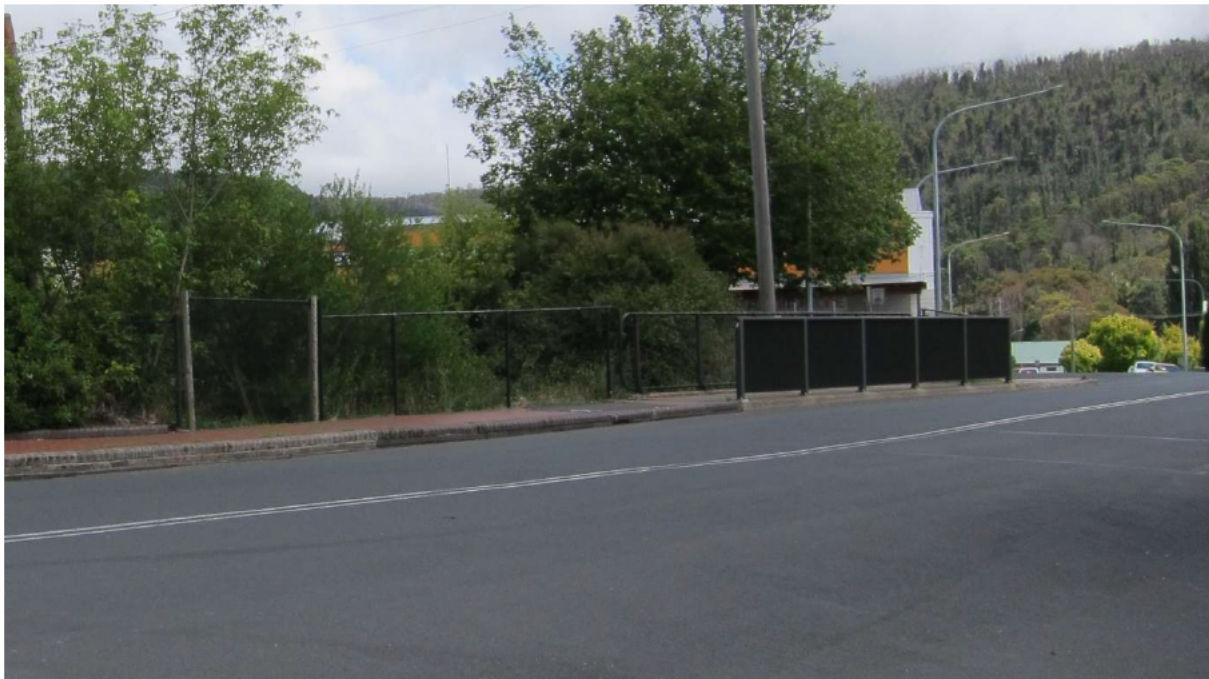
Figure 22. Pedestrian walkway and barrier on western side of overbridge, view north west (Source: Heritage Now 2023)
