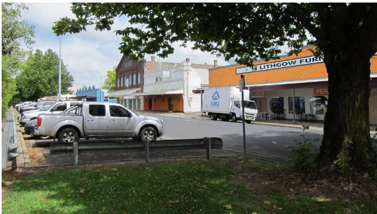
Figure 29. View north west from Work Area 1 at the intersection of Railway Parade and Bridge Street, toward the former Co-operative Store (centre of frame) (Source: Heritage Now 2023)
