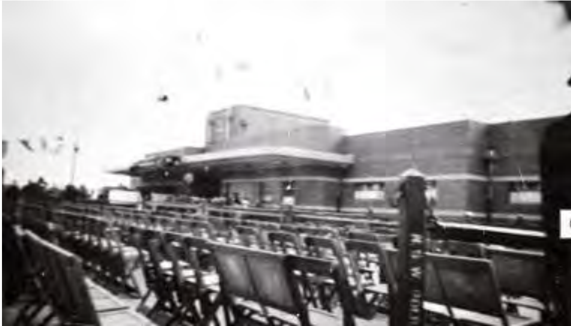
Figure 8: Photograph of the opening of the station in 1939 (Source: Sutherland Shire Library, Image No. MF006\MF006332).
