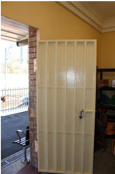
Figure 26: Storage room door.
