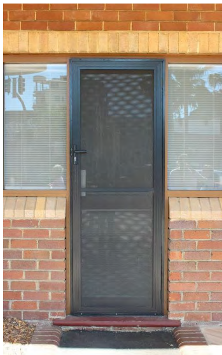
Figure 31: Entry to office showing modern aluminium windows and door.
