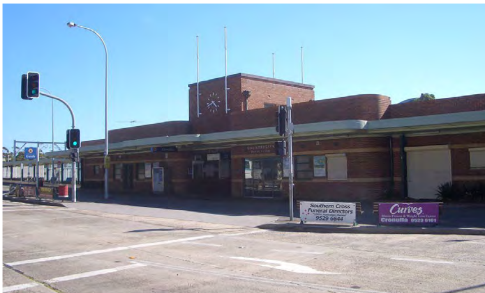
Figure 16: View of Cronulla Railway Station from Cronulla Street.
