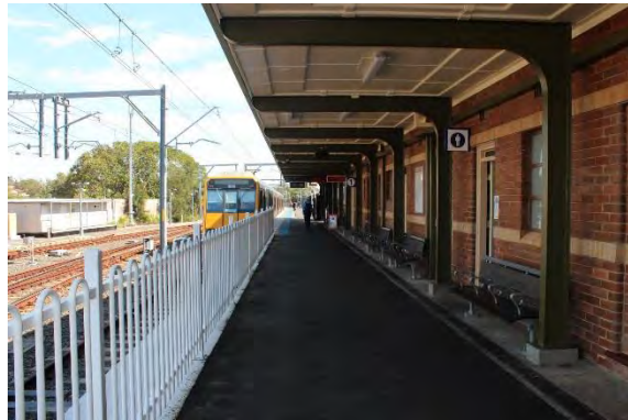
Figure 18: View along the platform.
