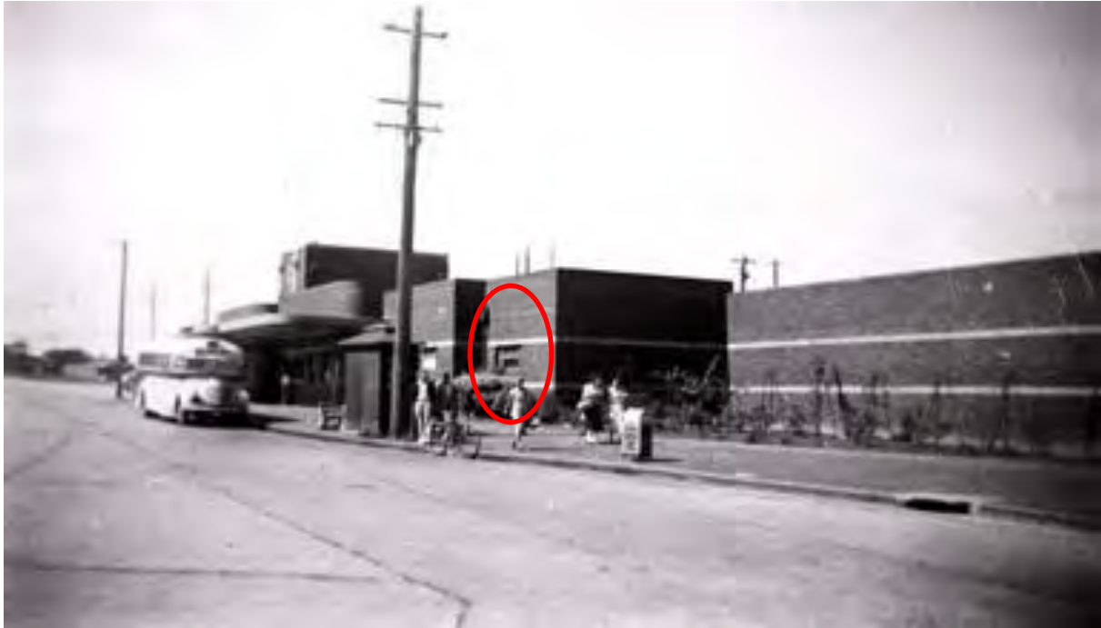
Figure 9: Cronulla Railway Station in 1948 showing the former window opening where an entry door is now located.
