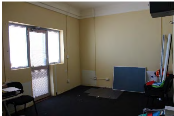
Figure 36: Interior of office.
