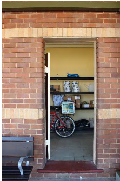
Figure 27: Entrance to store room, features original brickwork and doorway.
