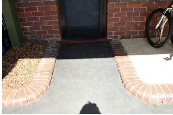
Figure 34: Paving to the front entry.
