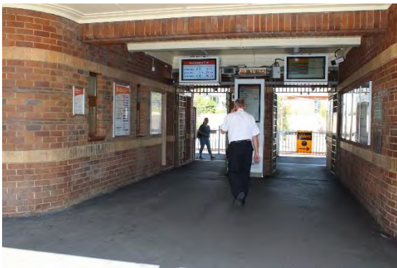
Figure 19: Entry to platform.
