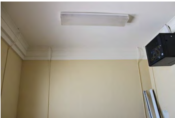
Figure 35: Interior of office.
