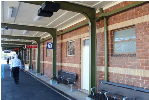
Figure 24: View of window (right) to store room from the platform.
