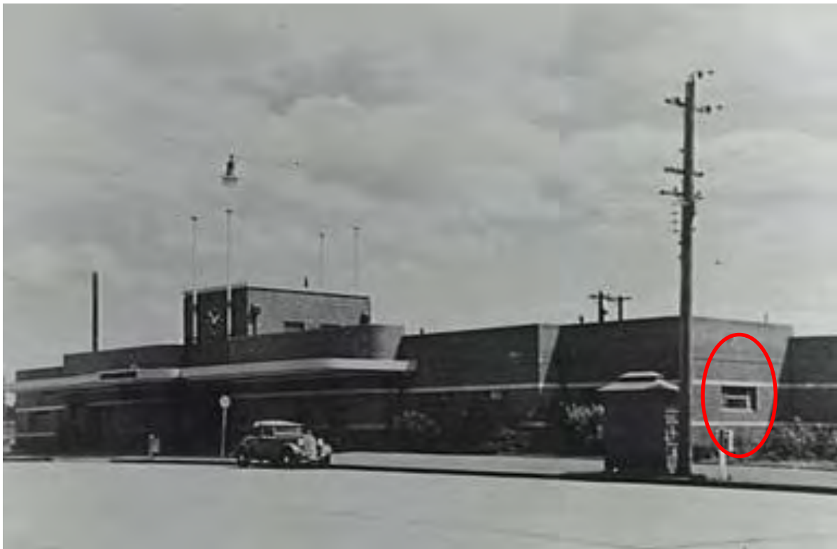
Figure 10: Cronulla Railway Station in the early 1940s showing the former window opening which was modified to a door in 1994.
