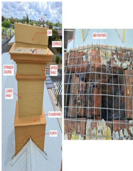
Figure 4-2 Chimney Notation Diagram
