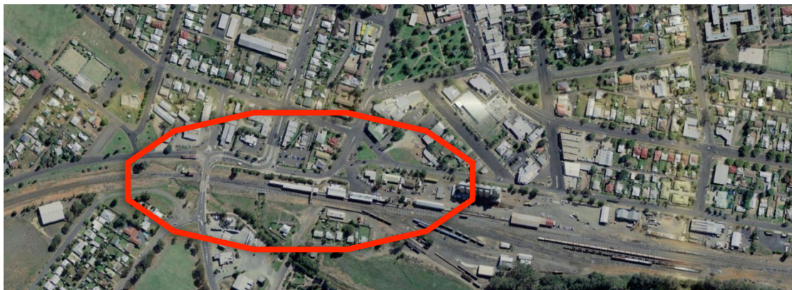
Figure 1 Parkes Railway Station
