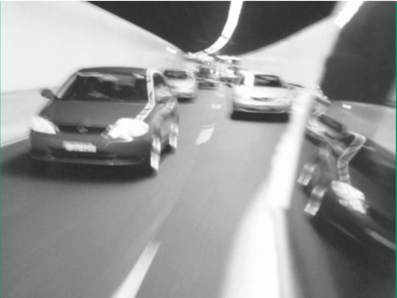
THE M5 EAST FREEWAY TUNNEL.
