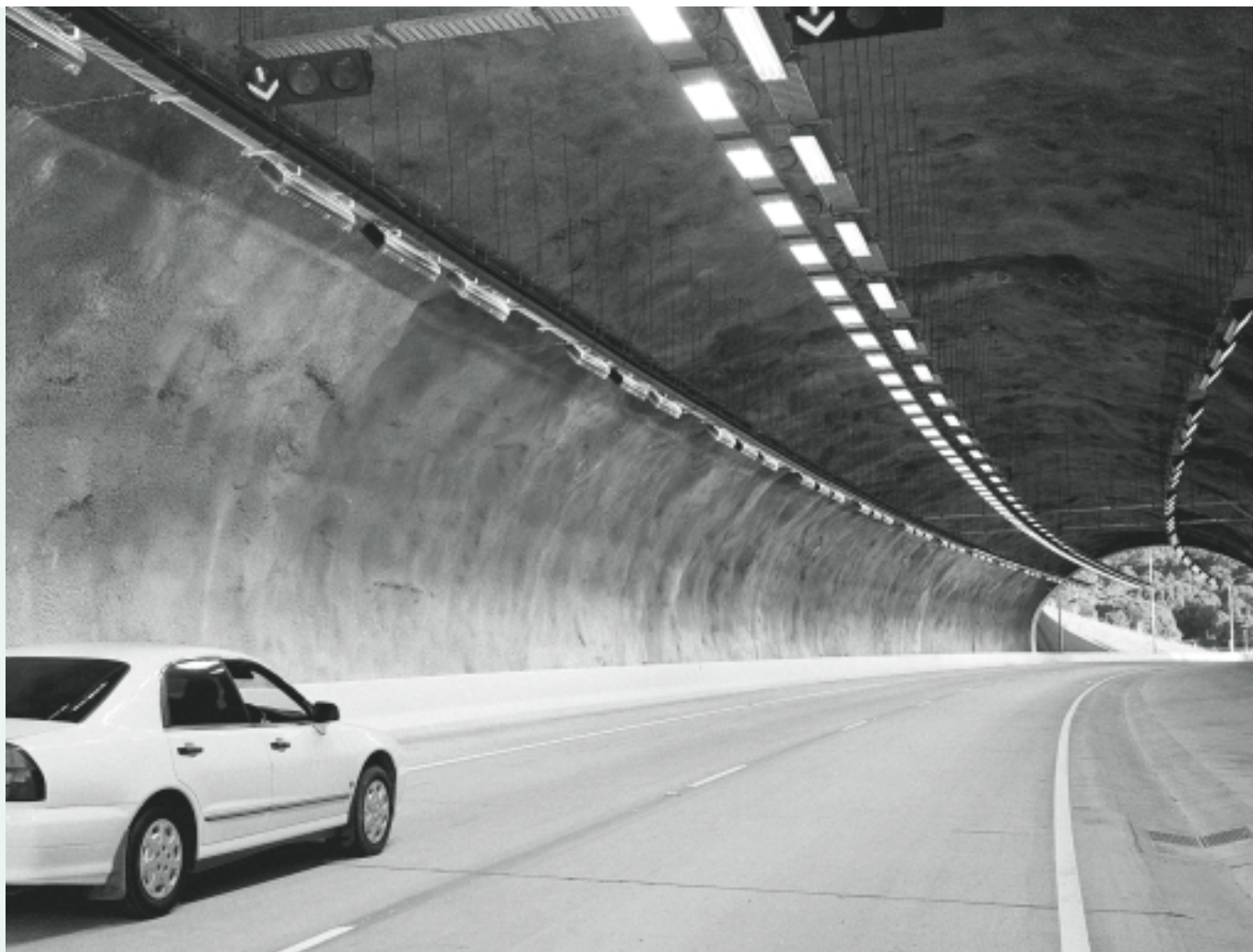
A SECTION OF THE YELGUN TO CHINDERAH PROJECT ON THE PACIFIC HIGHWAY.
