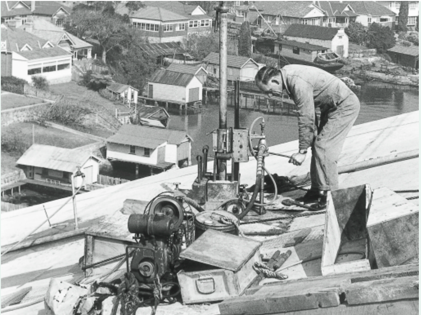
THE BUILDING OF GLADESVILLE BRIDGE (1960–1964).
