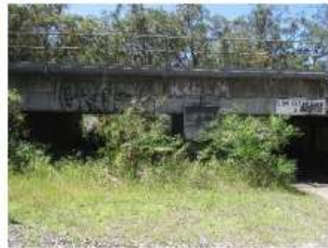
Figure 14. View east of bridge established between Vales Point and Morisset station.
