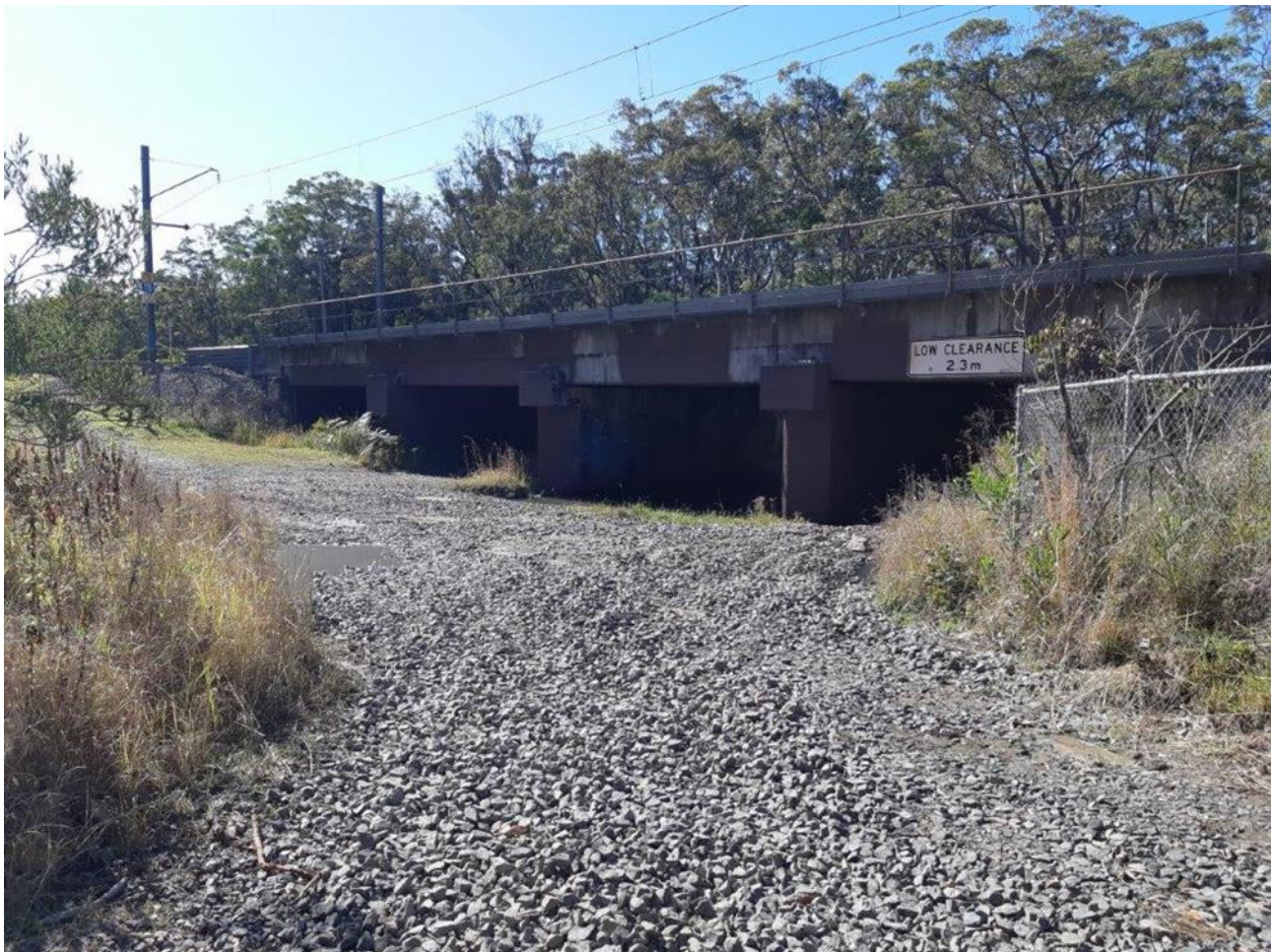
Figure 5-8: Pourmalong Creek and the Rail Bridge Crossing
