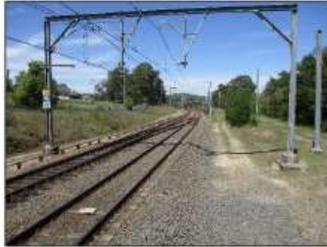
Figure 5. View south showing the cut into the sloping landform to establish Morisset Station.
