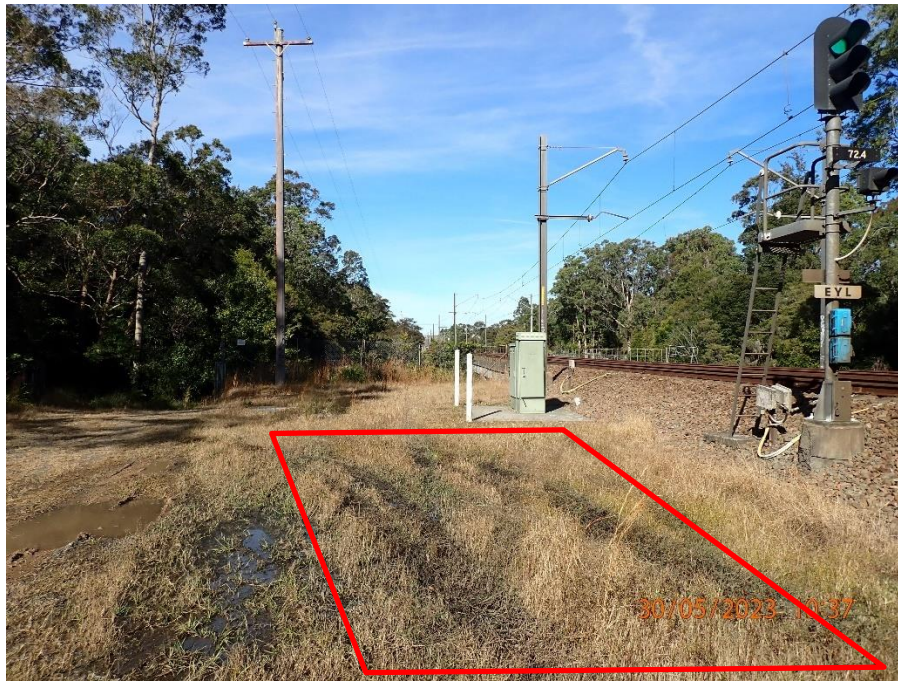
Image 05 – Approximate location of the MT1 structure
