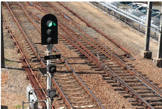
Figure 4-3: Standard track signal, Morisset
