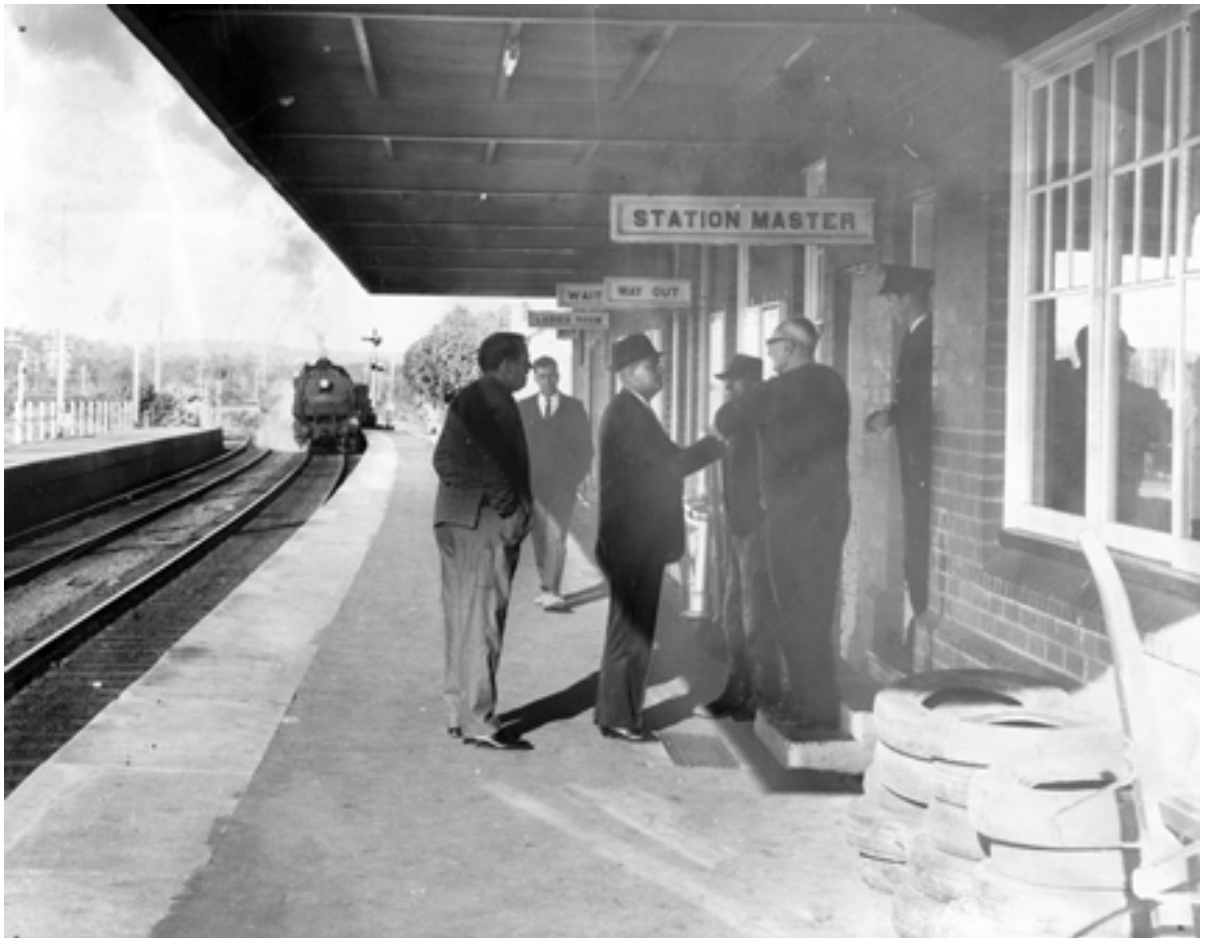
Figure 3-6: Morisset Railway Station (September, 1969). Newcastle Morning Herald, 1969. Newcastle Libraries, Hunter Photo Bank https://newcastle-collections.ncc.nsw.gov.au/library?record=ecatalogue.75393 Note relevant station elements which are no longer present: the signage above the doors, and the semaphore style signals (in the background near the locomotive) which have been superseded and long since removed.
