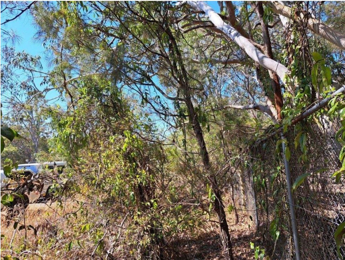
Figure 5-11 Overhanging tree limbs over boundary fence at Signalling Building MT29
