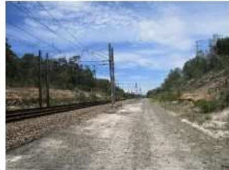
Figure 12. View south of cut into bedrock.
