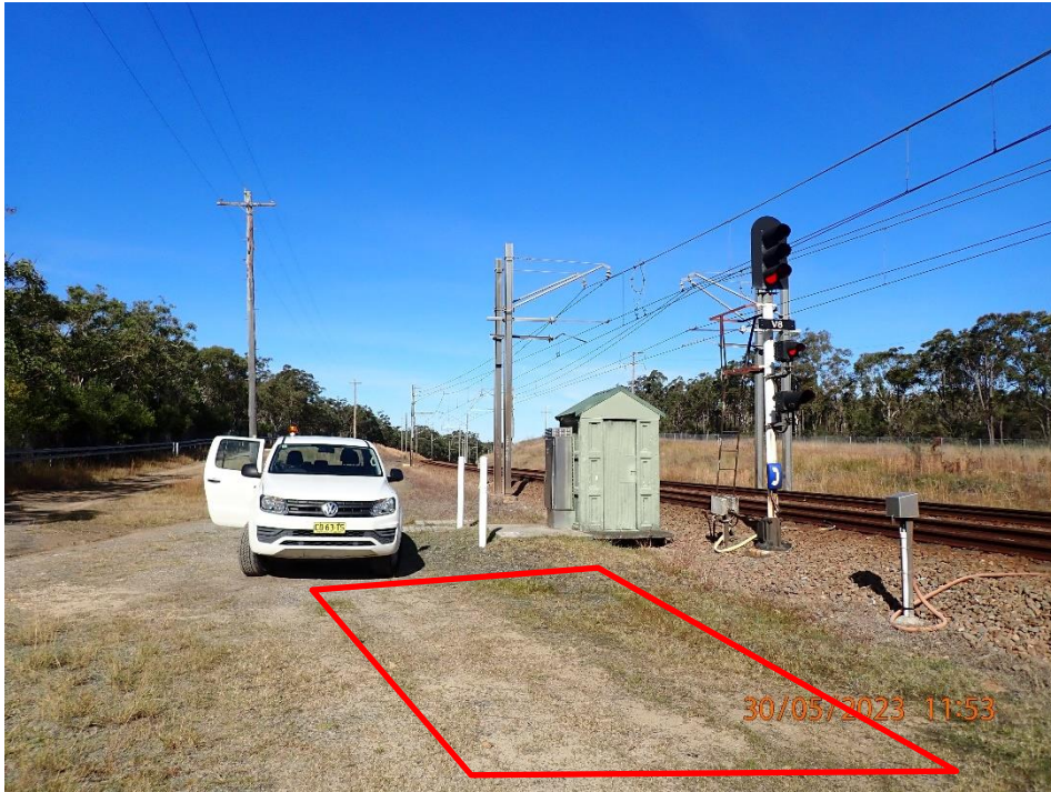
Image 13 – View of MT8 location in front of existing equipment shed.
