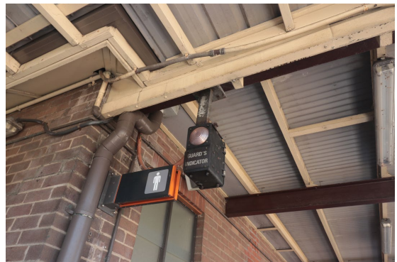
Figure 4-4: Standard guard's indicator with Fresnel lens
