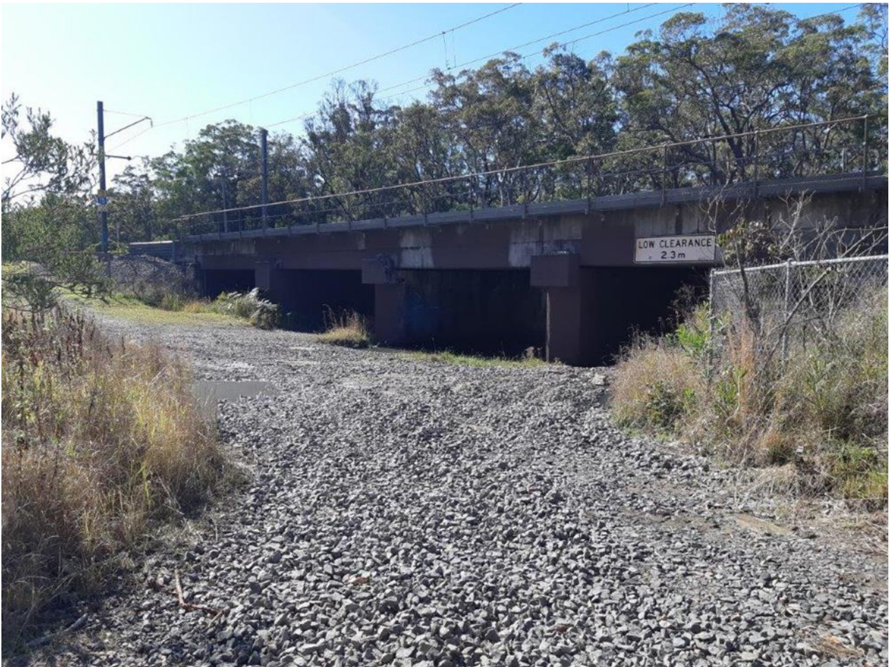
Figure 3–15: Bridge and gravel causeway over Pourmalong Creek, looking north east.
