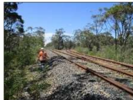
Figure 16. View south of artificial terrace landform established for the Vales Point Balloon Loop.
