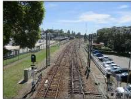
Figure 8. View north of existing signals and infrastructure immediately north of the Morisset Station.
