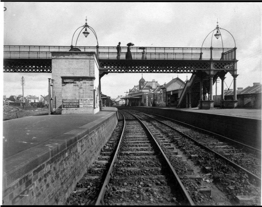
Figure 7: Railway bridge for passengers, Petersham, undated. Source: State Library of NSW collections file number FL8771104.
