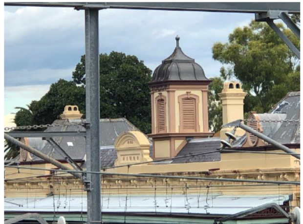
Figure 12: View of southern side of the roof (OCP, 2023)
