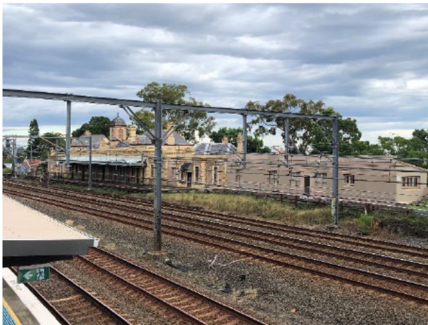
Figure 11: View of southern façade and roof from the platform (OCP, 2023)
