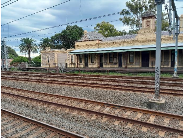
Figure 13: View of southern façade (OCP, 2023)
