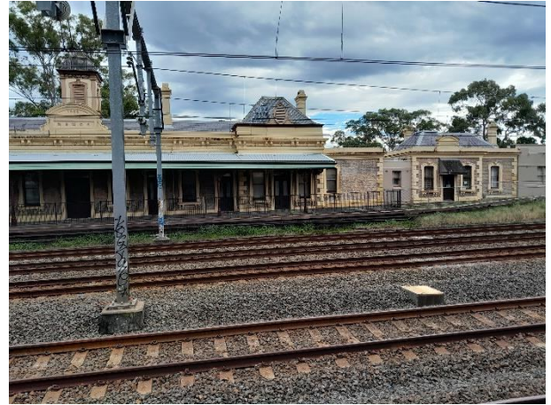
Figure 14: View of southern façade (OCP, 2023)
