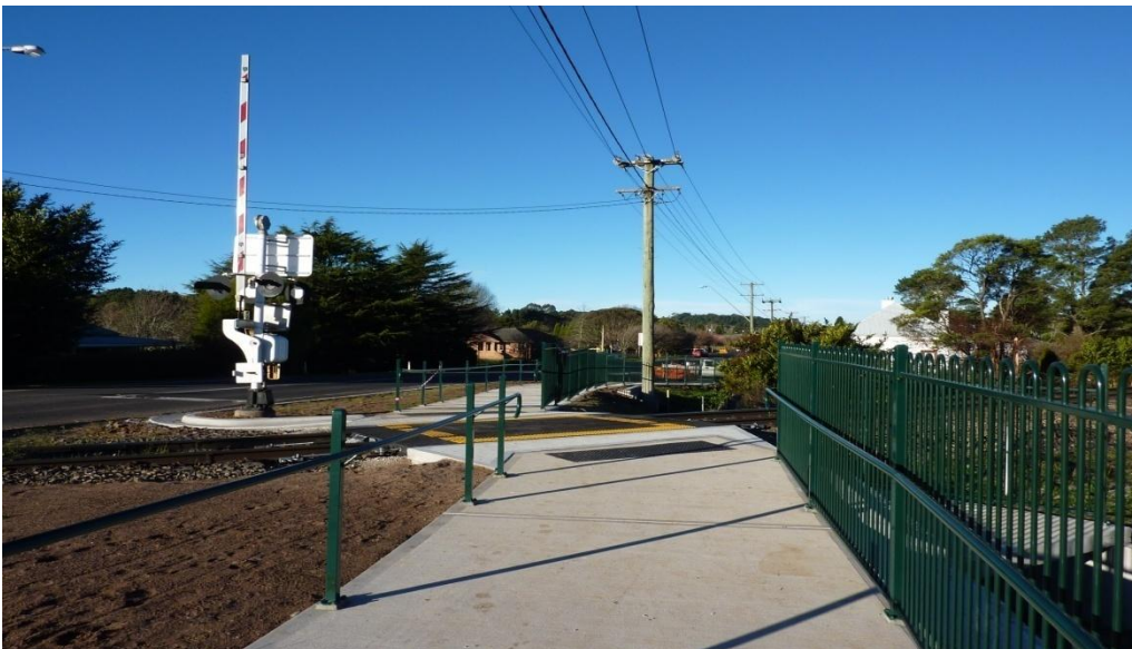
Figure 9 - Hoddle Street Level Crossing (Illawarra Highway), Robertson
