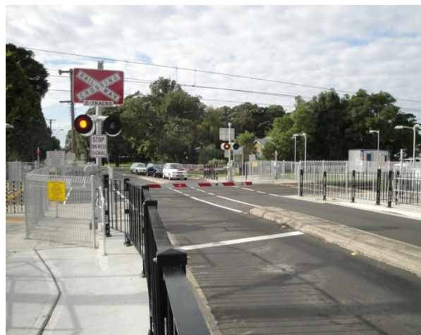
Figure 15 - Railway Street Corrimal - road crossing, pedestrian crossing
