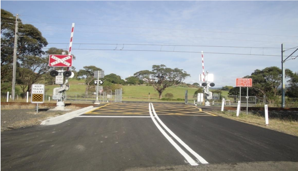
Figure 8 - Tip Road Level Crossing, Dunmore
