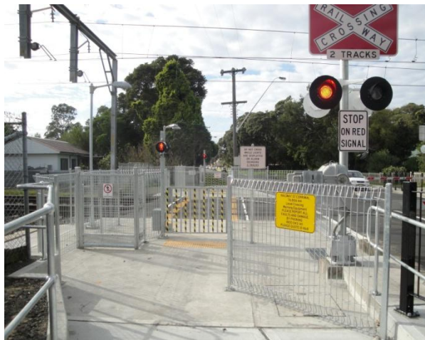
Figure 14 - Railway Street Corrimal - Up Sydney side
