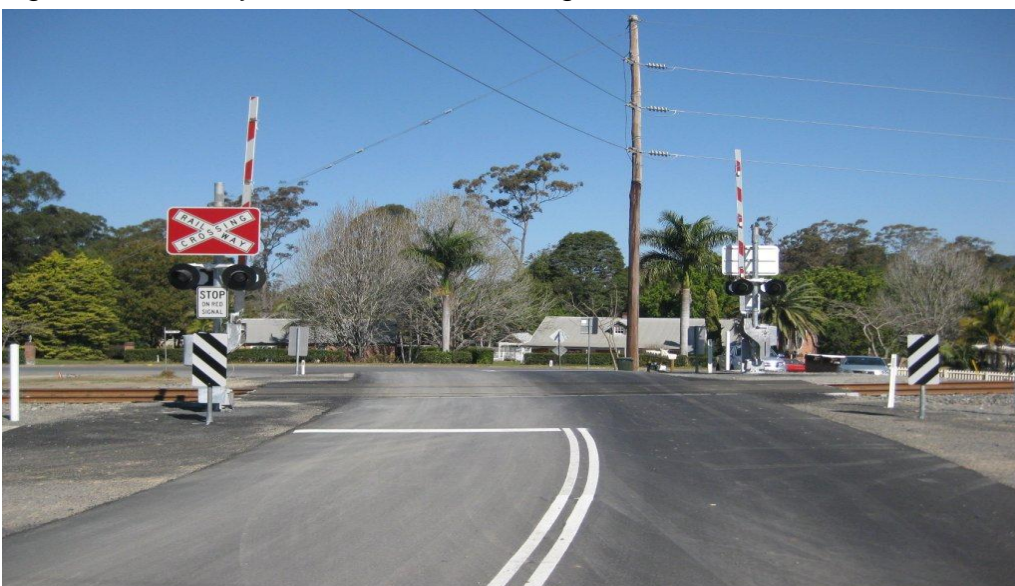
Figure 7 - Mackays Road Level Crossing, Coffs Harbour
