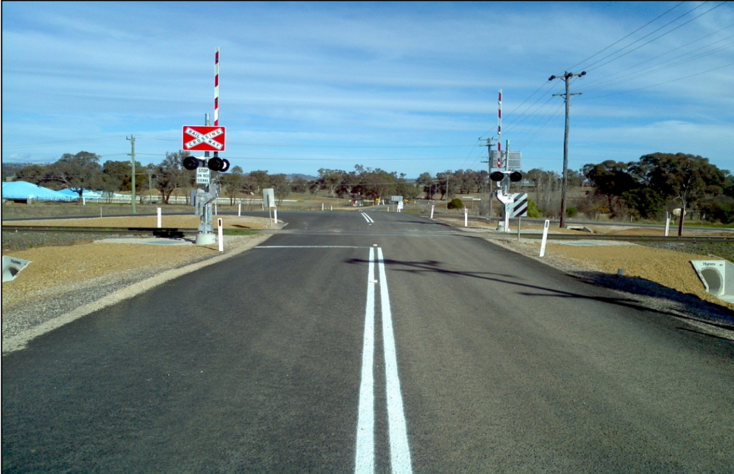
Figure 6 – Boree Street level crossing, Manildra
