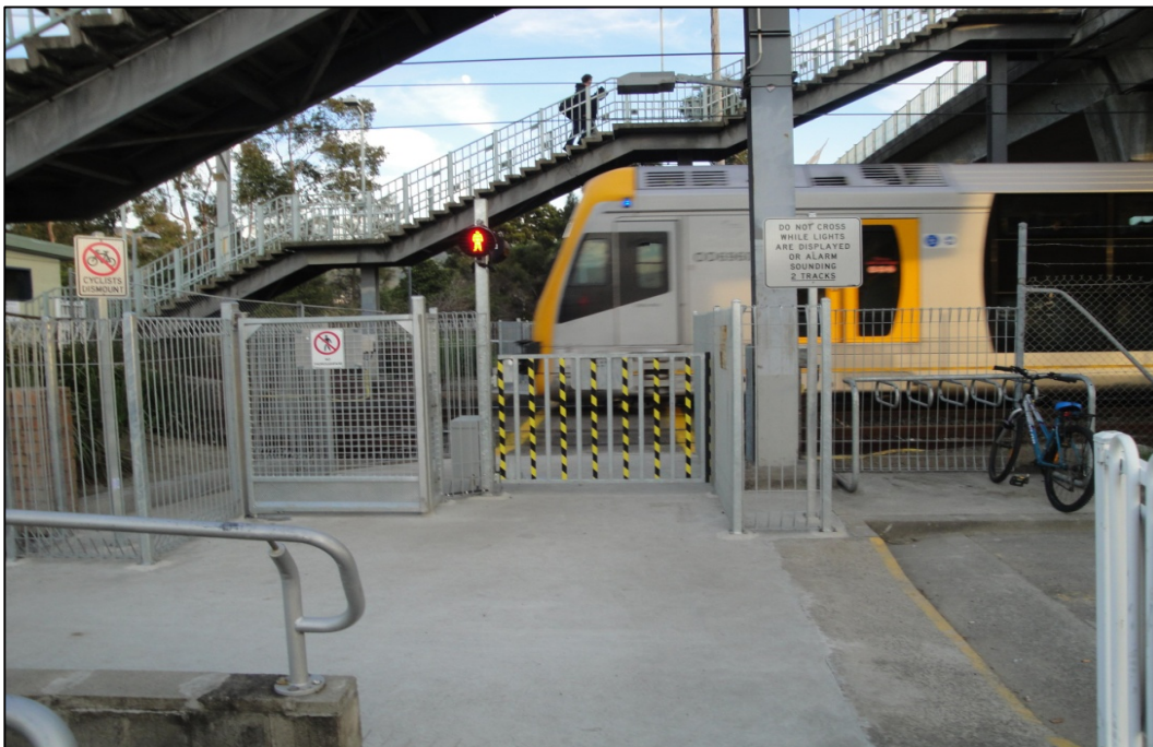
Figure 16 – Fairy Meadow Station Pedestrian Crossing
