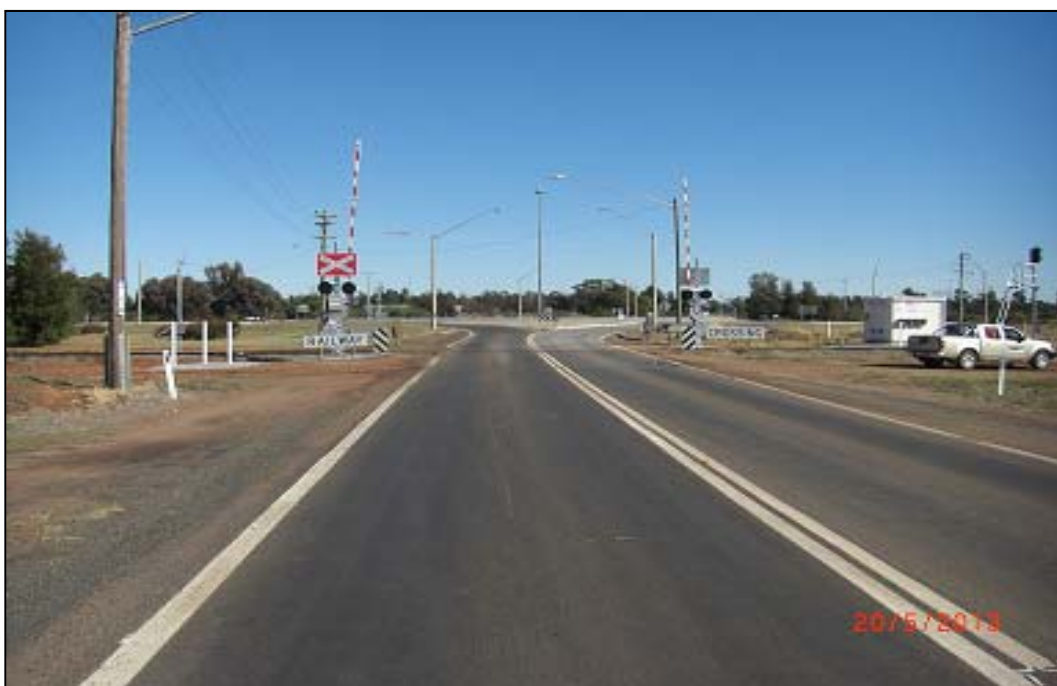
Figure 5 – Mid Western Highway level crossing, Goolgowi
