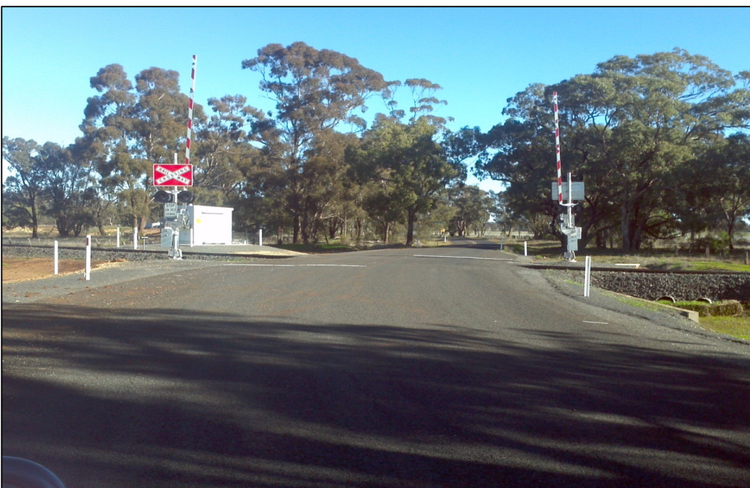
Figure 8 – Mogriguy Road level crossing, Mogriguy
