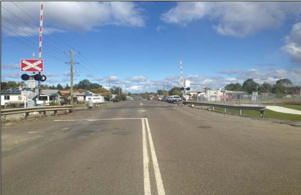
Figure 7 – Primrose Street level crossing, Wingham
