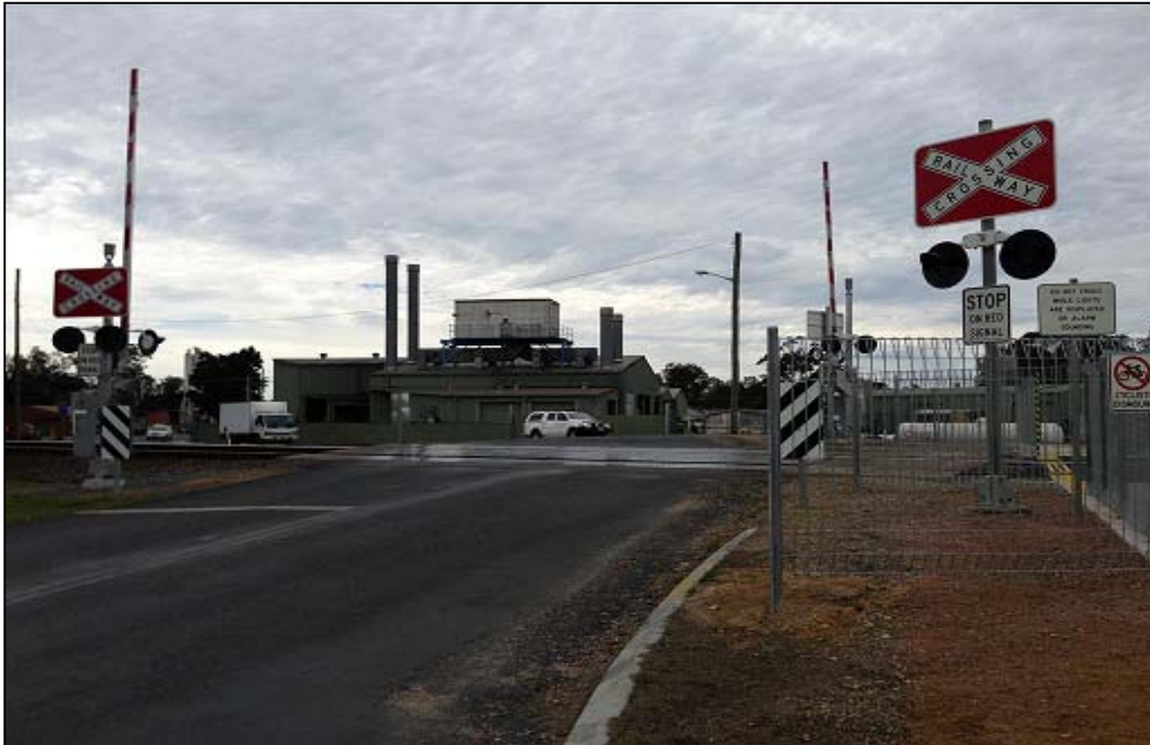
Figure 9 – Tilly Willy Road level crossing, Macksville
