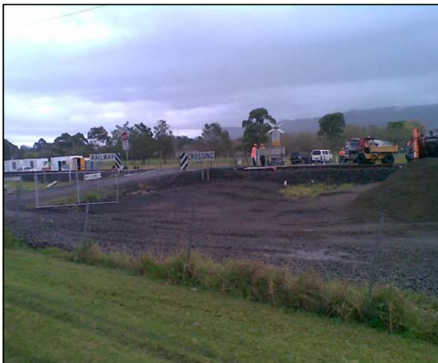
Figure 17 – Mullers Lane Berry Construction works
