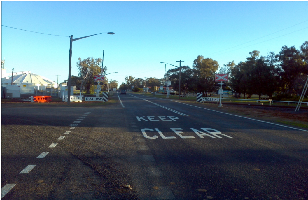
Figure 10 – Newell Highway level crossing, Gilgandra
