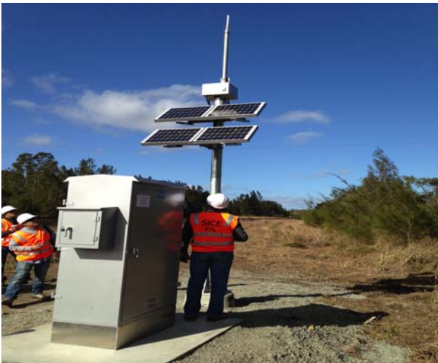
Sice Pty Ltd level crossing warning system installation in NSW
