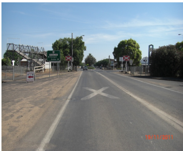
Dandaloo Road, Narromine (Before)
