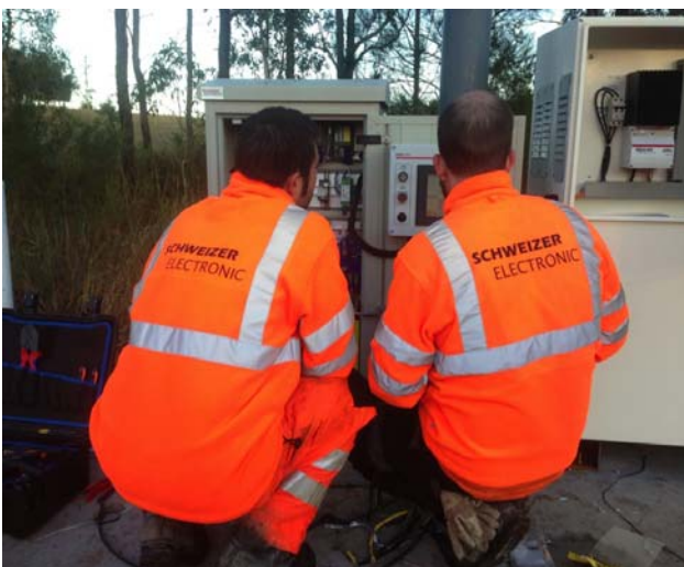
KH1 Pty Ltd Schweizer level crossing warning system installation in NSW
