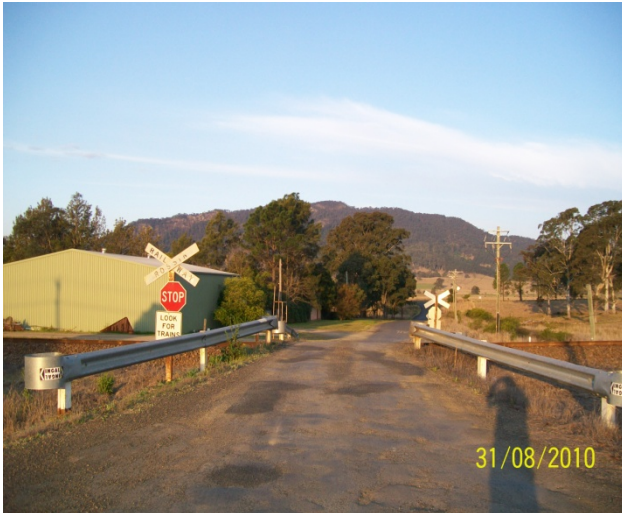
Phillips Street, Gloucester (Before)
