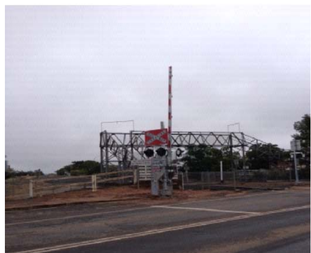
Dandaloo Road, Narromine (After)
