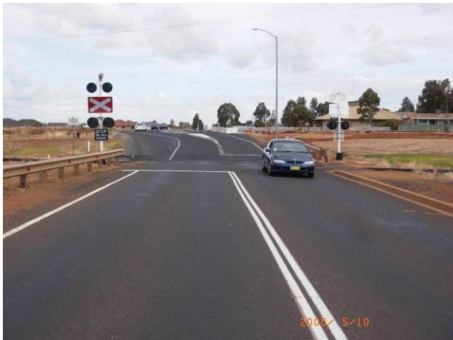
Sheraton Road, Dubbo (Before)
