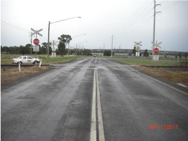
Yarrandale Road, Dubbo (Before)
