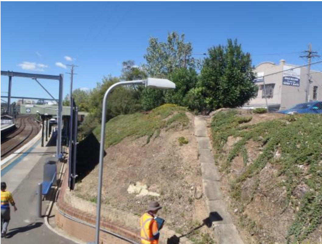
Plate 14 Embankment above platform 5 with prostrate conifer and garden areas above
