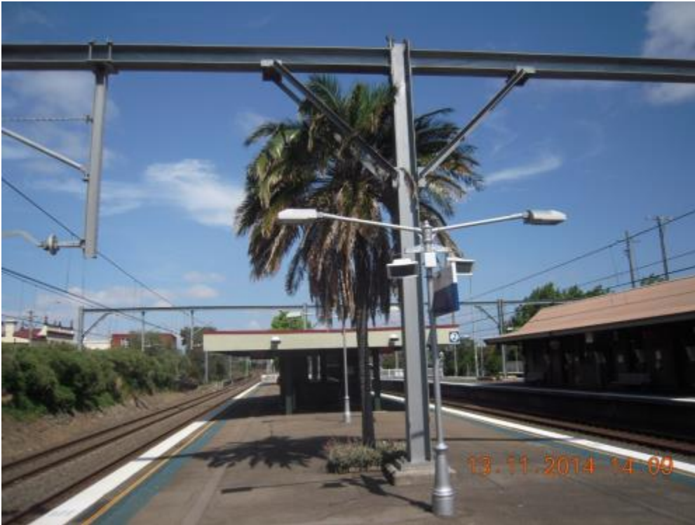
Plate 1 Heritage Listed Date Palm on platform 1/2 (tree 23)
