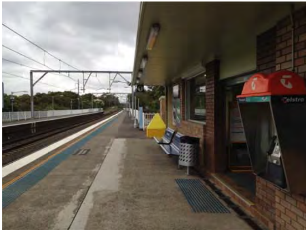
Photograph 9: Main Station Building
