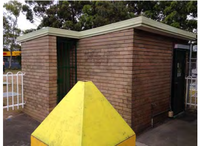
Photograph 8: Storage and Signalling Building
