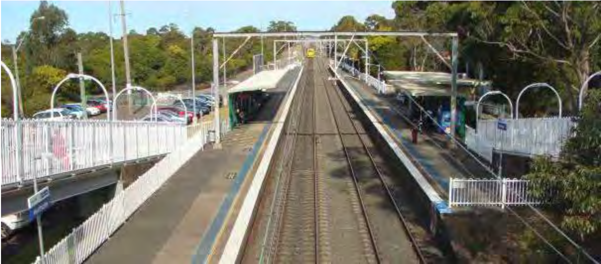
Image 4: View of the existing platforms looking south from the existing pedestrian overpass
