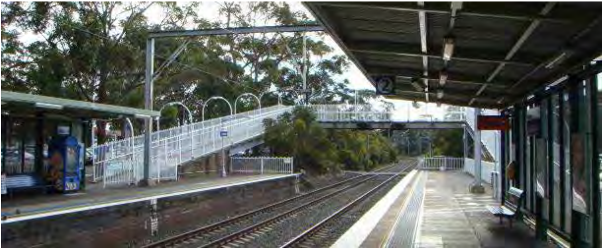
Image 3: View looking north from the eastern platform showing existing pedestrian overpass
