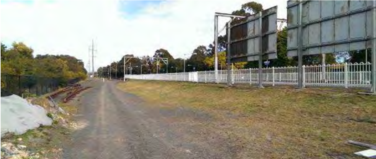
Image 7: View looking south of the proposed location of the extended eastern car park
